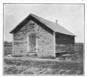
FIGURE 15.—An insulated frame potato-storage house used for storing second-crop potatoes. Morrill, Tex.
