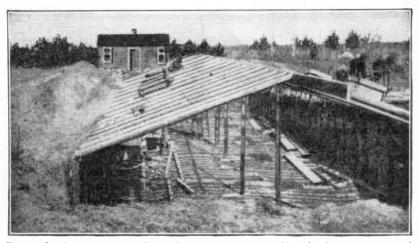
FIGURE 6.—A potato-storage house in course of construction, showing posts recessed in walls of earth and the method of placing ventilators in the roof. Jerome, Idaho
