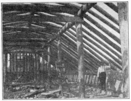
FIGURE 9.—Interior view of a potato-storage cellar with side and end walls of stone, showing the type of roof construction used. Greeley, Colo.
