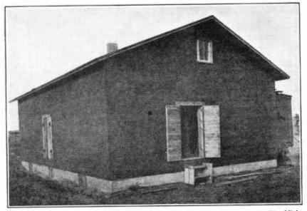
FIGURE 16 .- An insulated frame potato-storage house with a cellar. Greenville, Mich.
