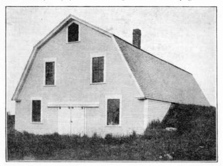
FIGURE 17.--A potato-storage house in Maine, showing a central driveway entrance into the lower or basement portion. The end entrance is more commonly used than the side entrance, especially in the larger structures
