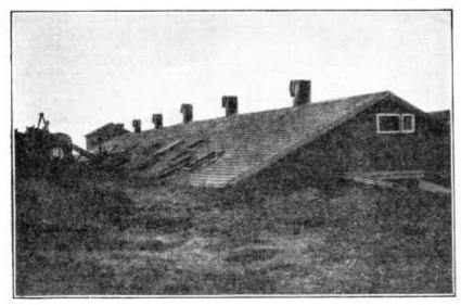
FIGURE 4.—A potato-storage cellar with water-tight roof, showing openings in the roof through which the tubers are spouted into the cellar. Sabin, Minn.
