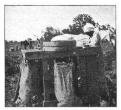
FIGURE 15.—The sizer or grader used hy Texas potato growers.
