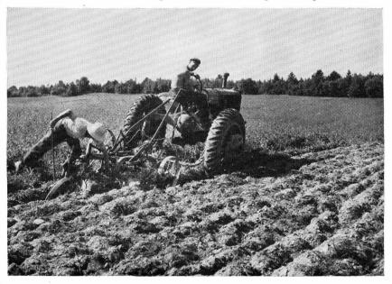
plowed more than an inch deeper than the plow depth. A 14-inch plow or larger is necessary to do a good job of plowing for potatoes. If much trash is to be turned under, plows with 16- and 18-inch bottoms and with a large clearance are needed. Fields with a decided slope should be strip-planted, and in most cases the plowing should be done in very late fall or in the spring to prevent undue erosion.
