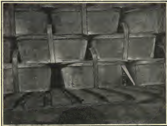
How Some of the Damage Begins.
