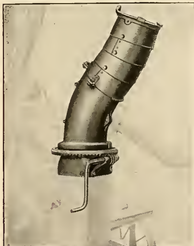
The above illustrations show the extremes to which the blower pipe can be raised or lowered
