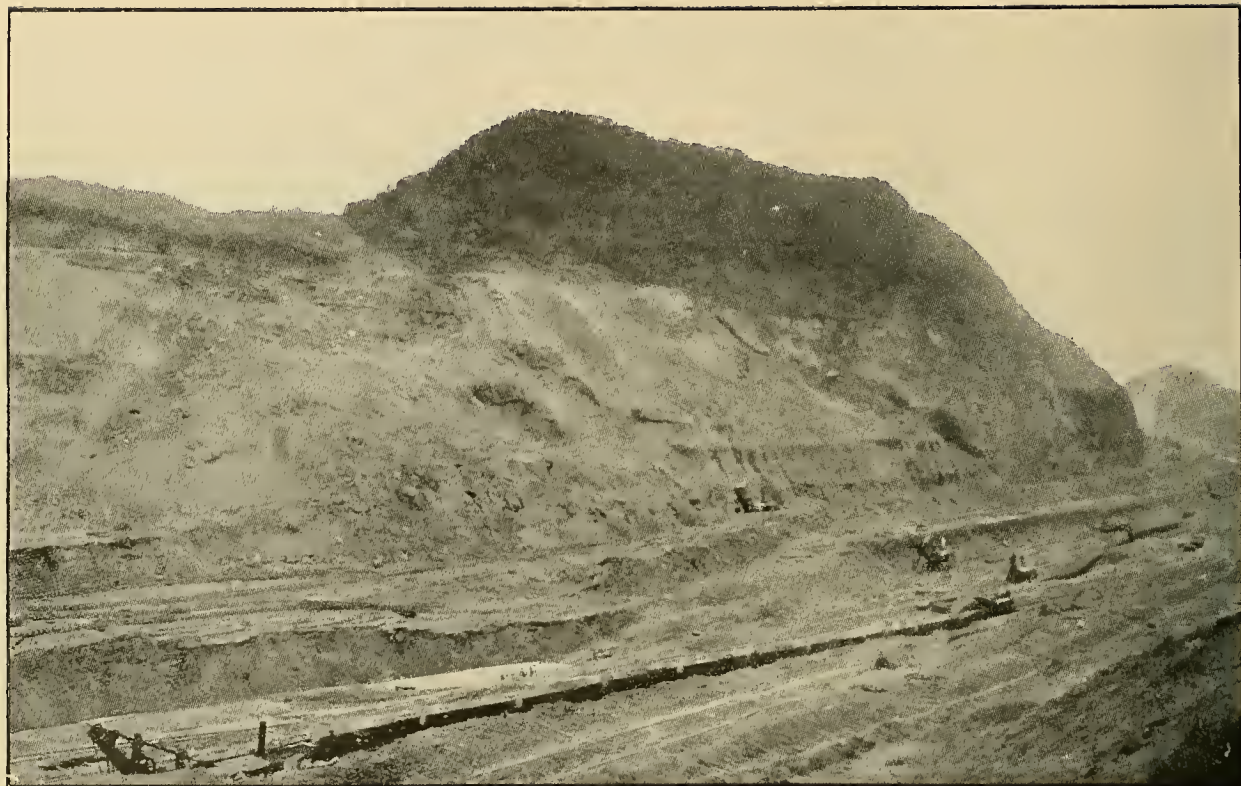
Culobra Cut, Culobra. Break in East Bank of Canal. Amount of Material Involved, 320,000 Cubic Yards. The Train Shown in Foreground Is About 35 Feet Above the Bottom, or at Elevation +75. Photographed February 11, 1912.
