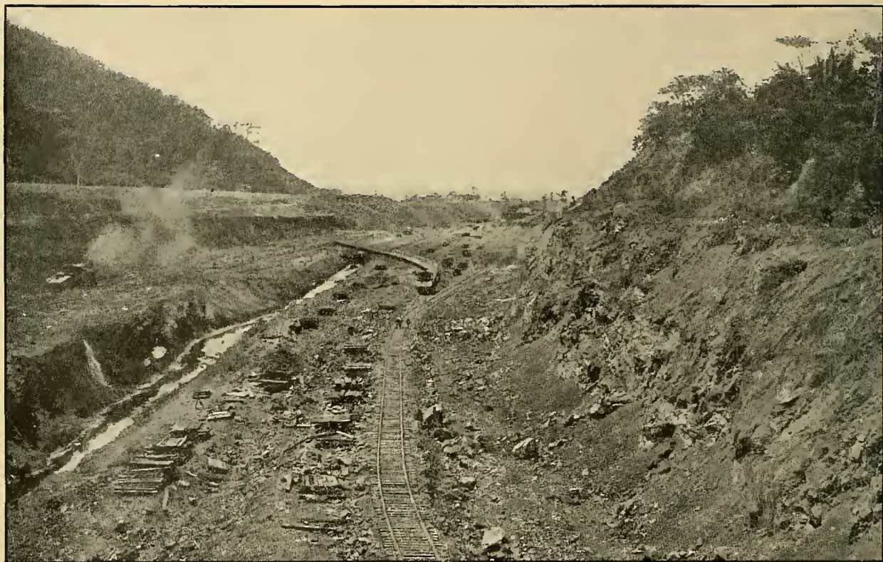
Culebra Cut, South End, Looking South from Bridge 57½ and Showing the Partly Completed Anchorage Basin North of Pedro Miguel Lock. Train Is on Completed Bottom of Canal, Elevation +40. Photographed June, 1912.
