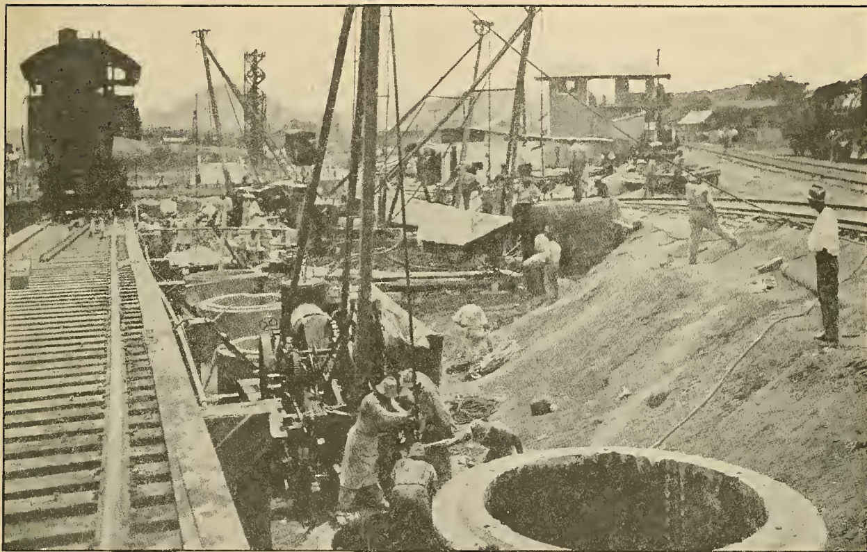
Miraflores Locks. Sinking Caissons for Foundation of North Approach Wall, Looking North, June 14, 1912.
