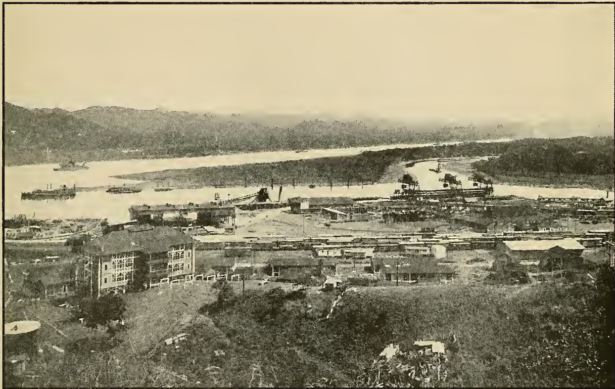
General View of Balboa Terminal Site, Looking North, June, 1912.
