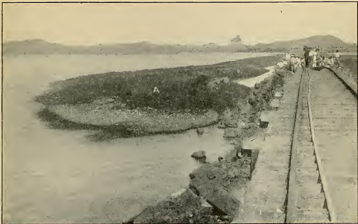
South End of Naos Island Dump, 4,000 Feet from Island. Center at "A" Is 80 Feet from Track and 25 Feet Above the Original Bottom. Elevation of Trestle, +14. Photographed in December, 1911.
