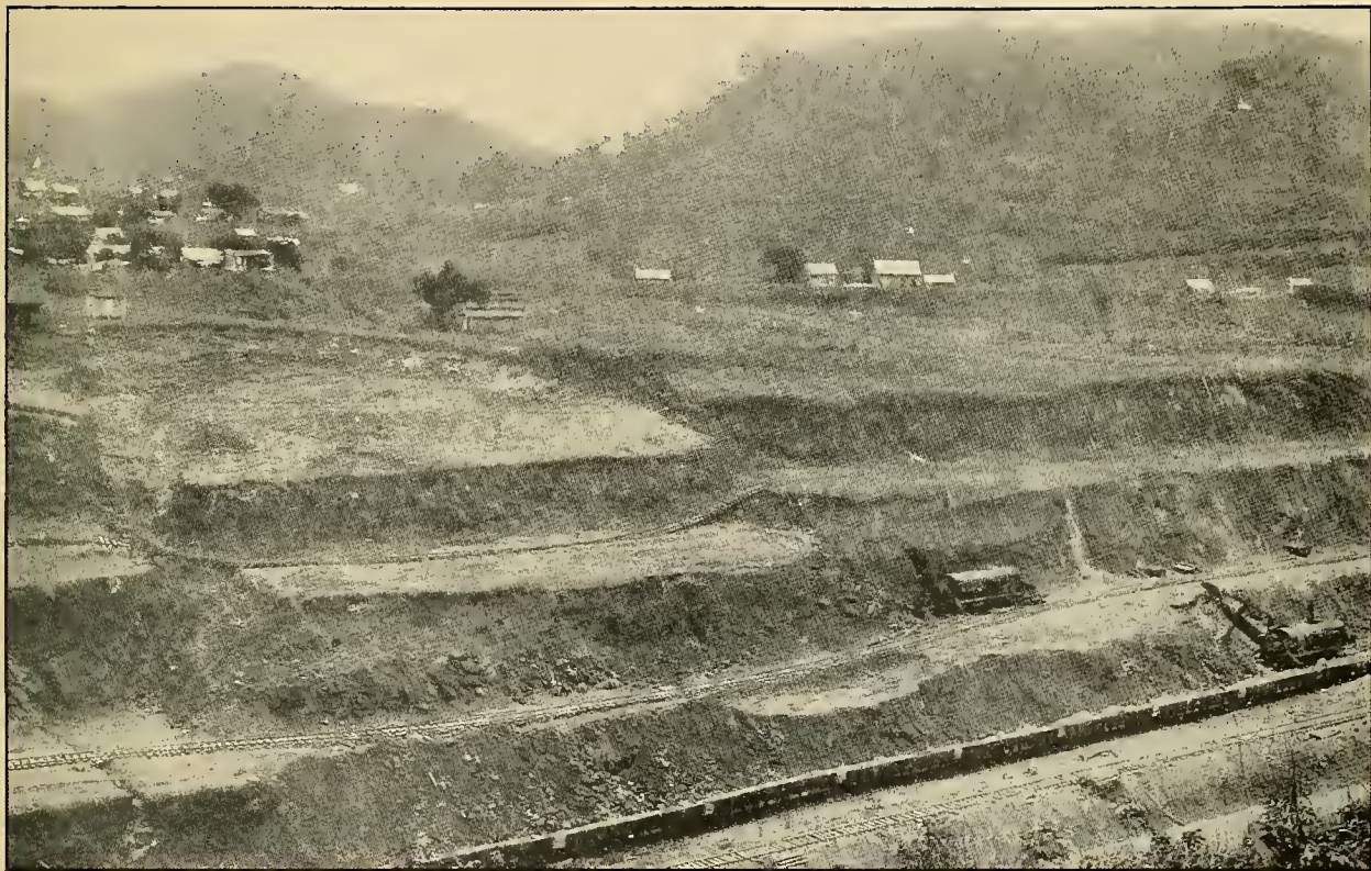
Slide in East Bank of Canal Near Cucaracha, June, 1912. This Illustrates One of the Difficulties with Which the Engineers and Construction Department Have Had to Contend.
