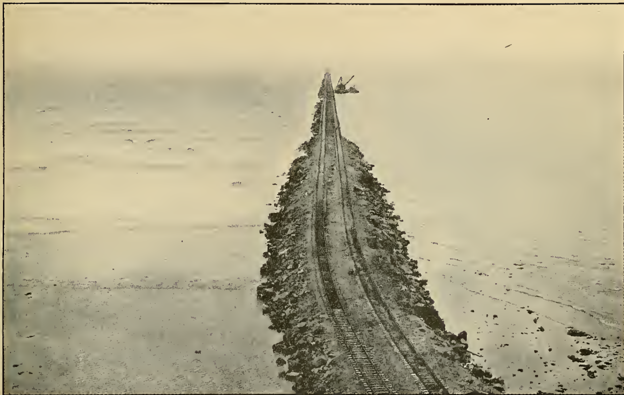
West Breakwater, Looking Seaward from Toro Point, Showing Dredge at Work Placing Rock on Face of Breakwater. Photographed June, 1912.
