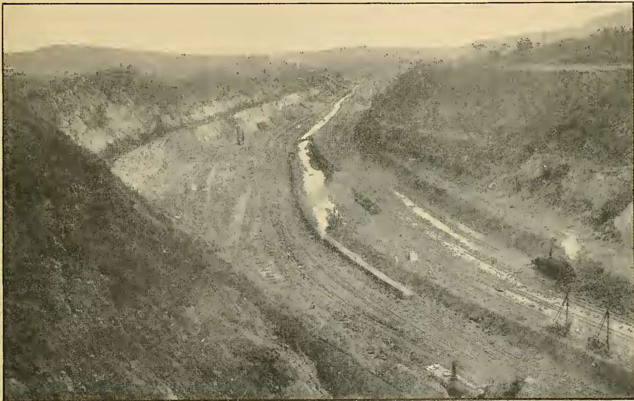
Culebra Cut Looking North from Cunette. The Two Shovels Shown in the Foreground Are Working on the Bottom, Elevation +40. The Water Standing in the Center Drainage Channel Is About 6 Feet Below the Bottom, Elevation +34. Photographed in June, 1912.
