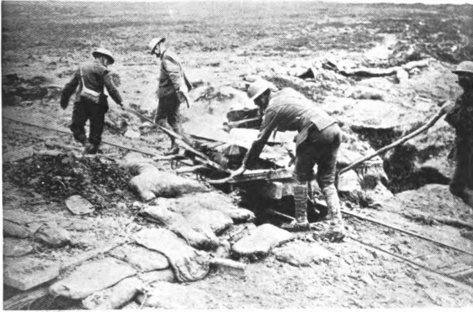
Narrow gauge construction
