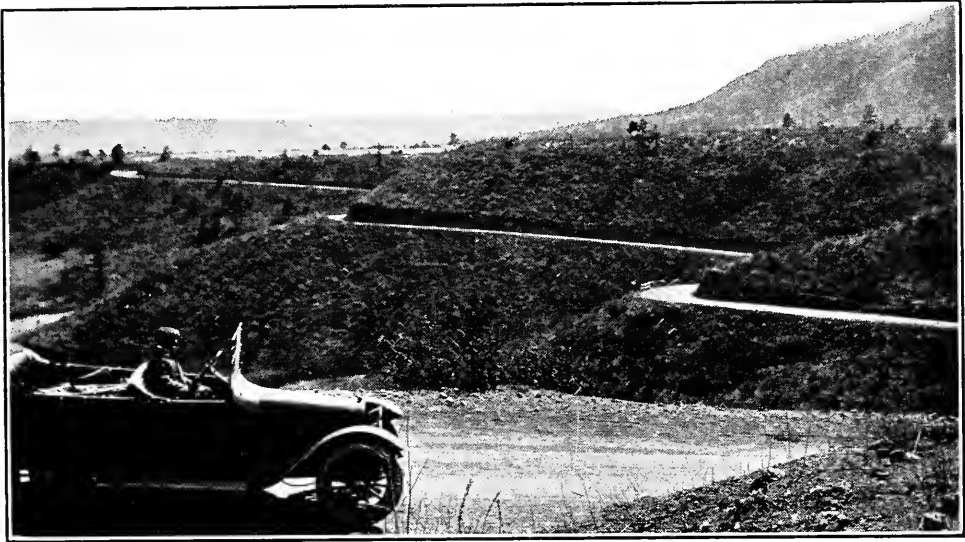
FIG. 41.—Alignment following grade contour closely (New Mexico).
