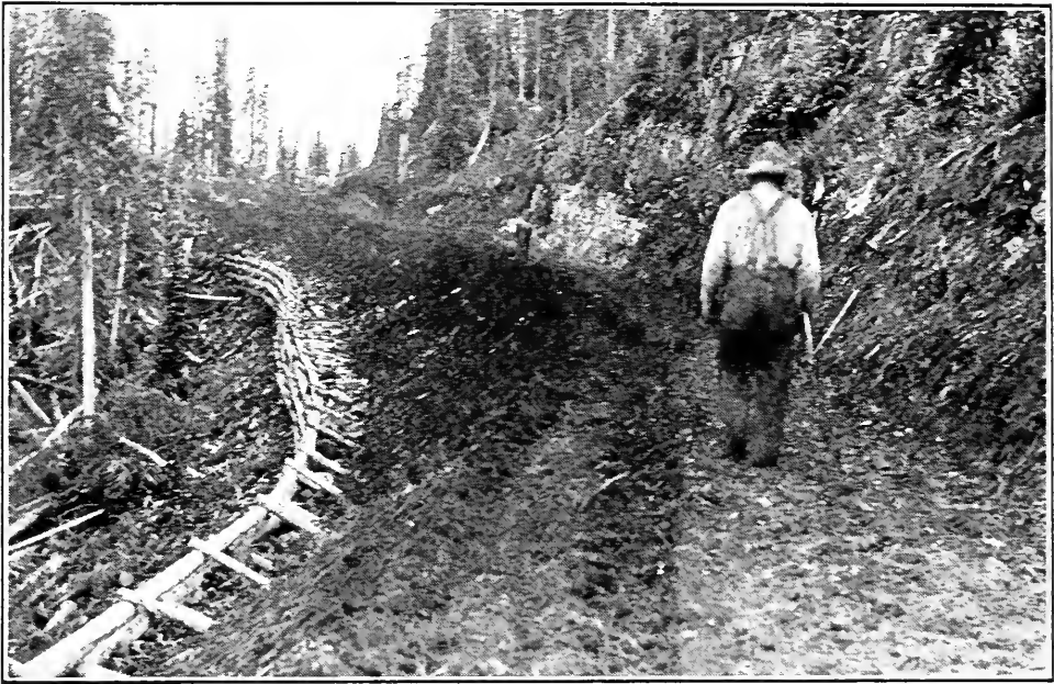
FIG. 81.—Temporary timber cribbing to hold fill.
