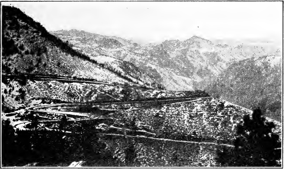
FIG. 43.—First class switchback design. Note flattening of grades on sharp turns.
