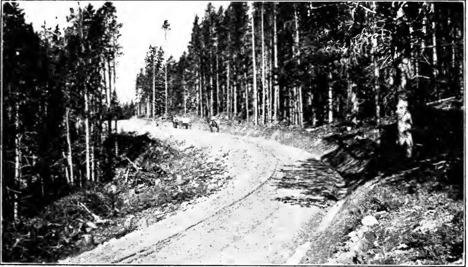
FIG. 39.—Example of first class side hill alignment. Also note liberal width of clearing to increase sight distance and to permit the sun to reach the road and melt snow.
