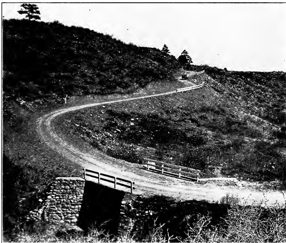
FIG. 31.—Balanced side hill section.
