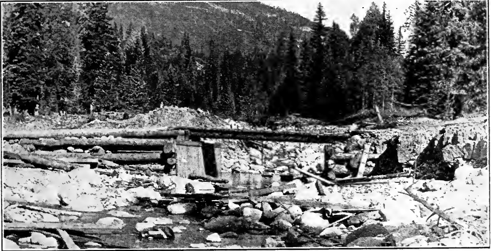
FIG. 109.—A crude log stringer bridge. Pioneer road work.
