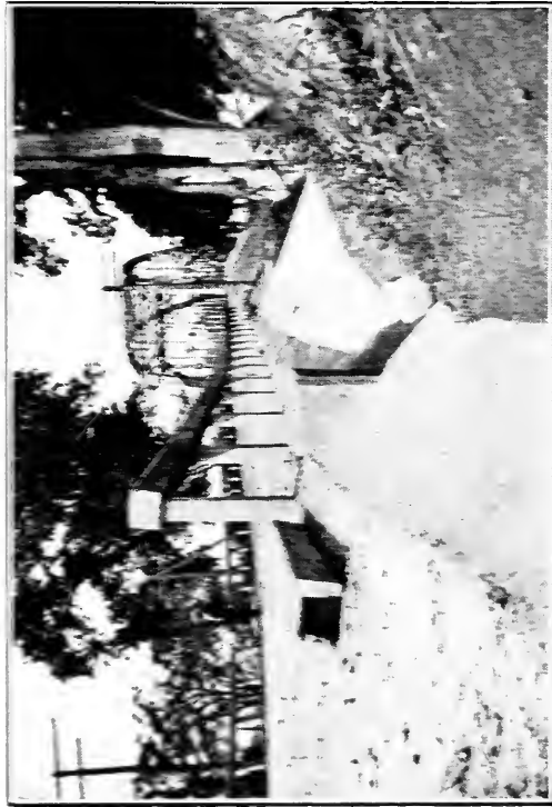
FIG. 101A. In times of high water this road is covered to a depth of 6 to 7 ft. Note the low water culvert, concrete shoulders to prevent scour, and concrete guard rail protection.
