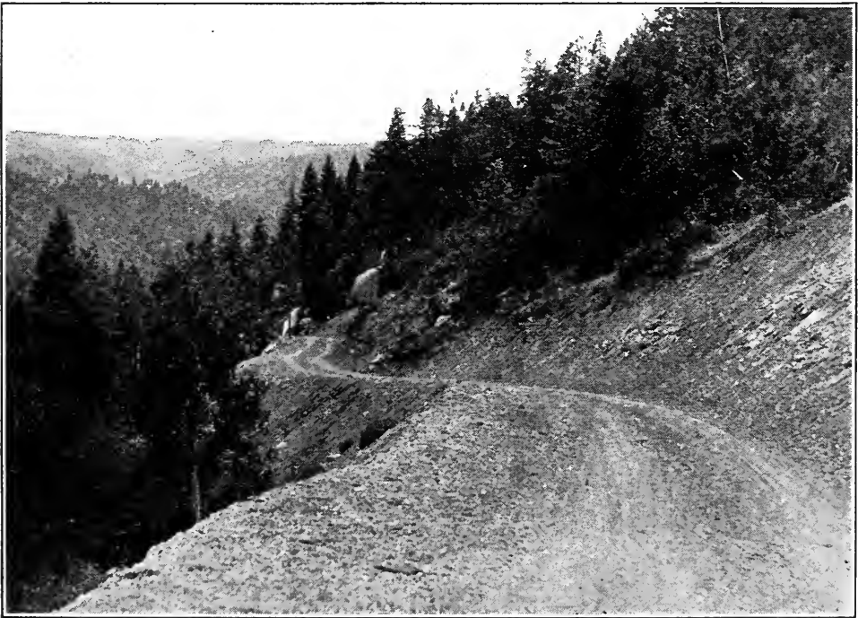
FIG. 40.—Example of ordinary side hill alignment.
