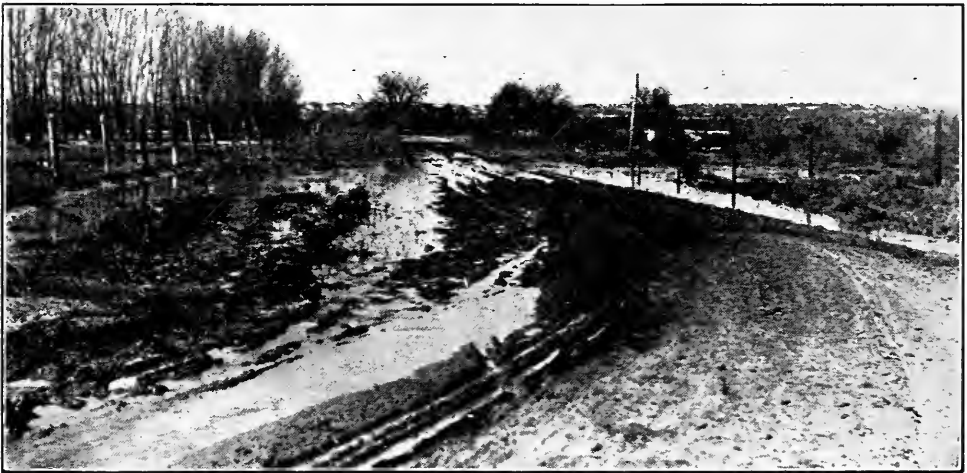
FIG. 90.—Undrained road conditions (Wyoming).
