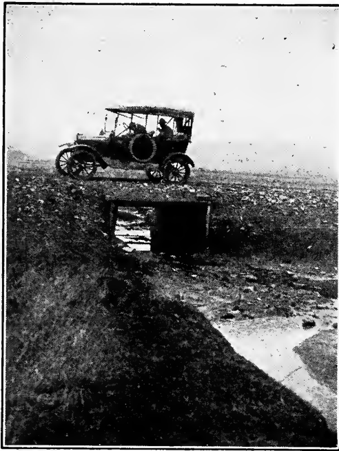
FIG. 91.—Temporary timber box culvert (Utah).
