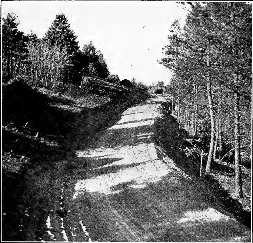
FIG. 73.—Good example of the “one way crown” section. Note also the careful clearing.
