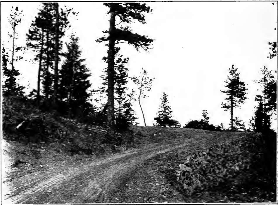
FIG. 46.—Retaining wall switchback construction.
