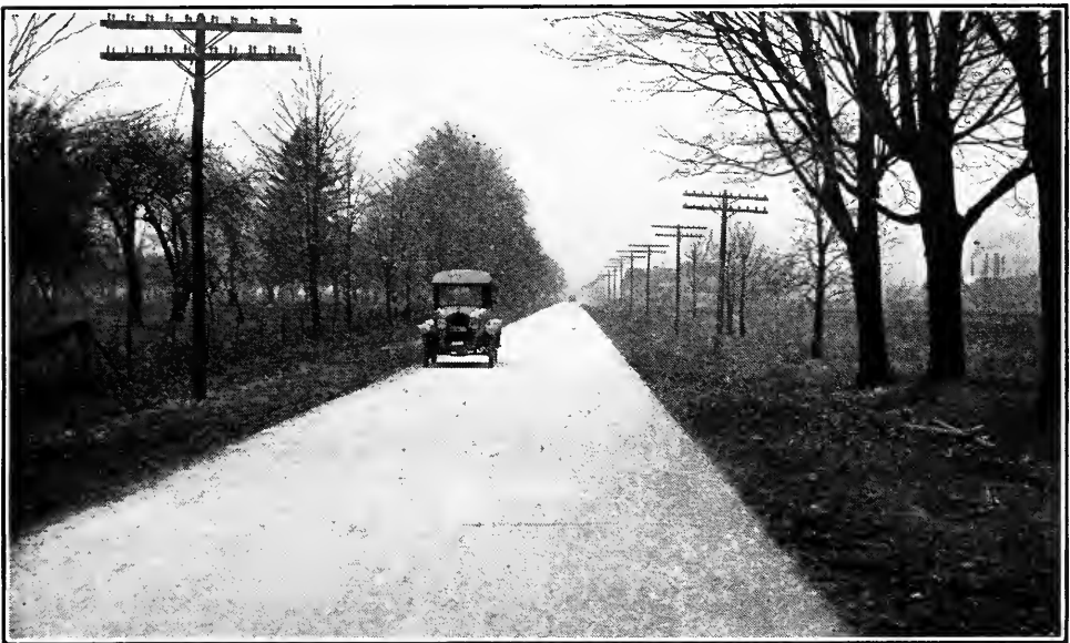
FIG. 6.—Typical rigid pavement highway (Industrial District Ohio). Note the shallow ditch which adds to the safety of traffic.
