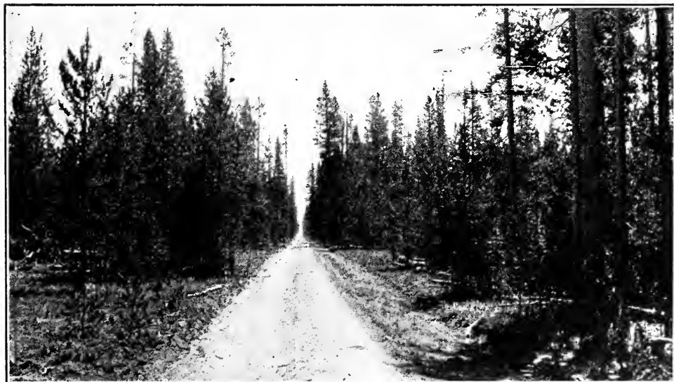
FIG. 80.—Simple turnpiking in easy location Targhee national forest (Idaho). Note the comparatively narrow width of clearing for small Jack Pine growth.
