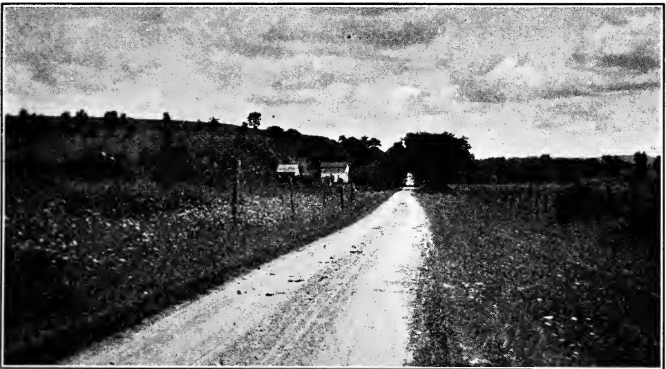
FIG. 4.—Typical single track gravel road (New York state). Very satisfactory for local traffic in agricultural districts. (The third stage of progressive improvement.)
