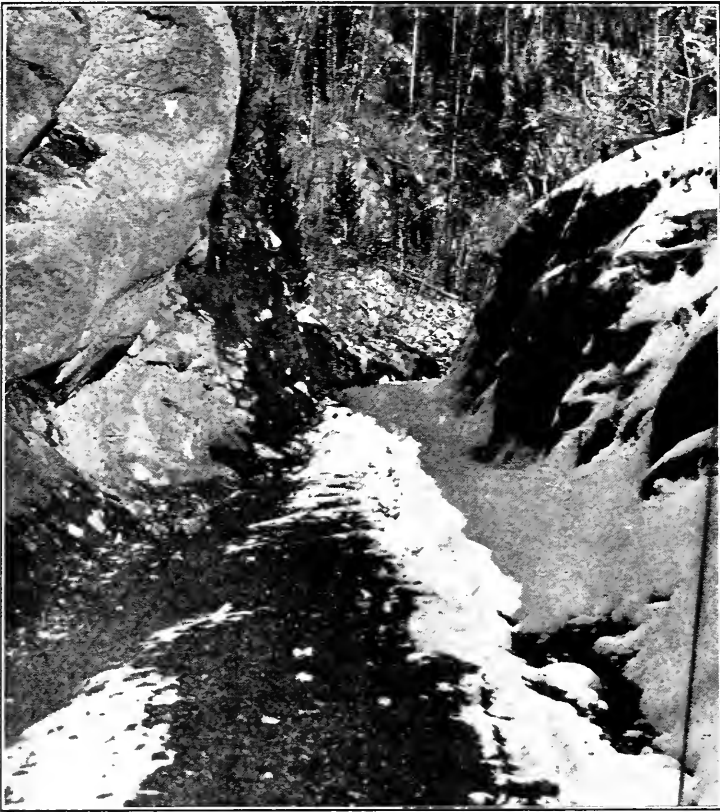
FIG. 77.—Narrow single track through cut section.
