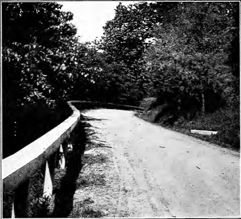
FIG. 48.—Banked curve on high class road protected by substantial concrete guard rail.
