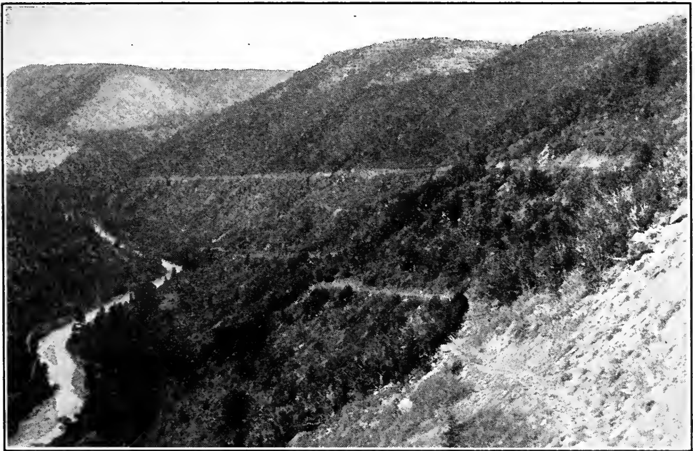
FIG. 17.—Example of engineering grade reduction. Pack trail in foreground. Newly located wagon road to the right and above. U. S. forest road project.
