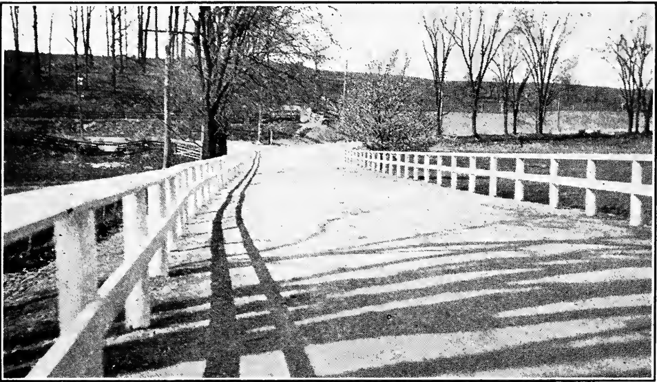
FIG. 37.—200 ft. radius curve in background on 3 per cent. grade. Serves traffic well. This road is a State Route in New York State carrying approximately 1500 vehicles per day in summer.
