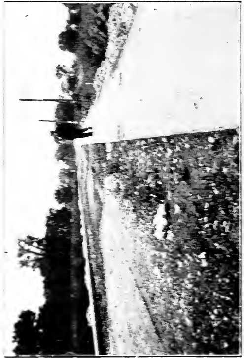
FIG. 101A. In times of high water this road is covered to a depth of 6 to 7 ft. Note the low water culvert, concrete shoulders to prevent scour, and concrete guard rail protection.
