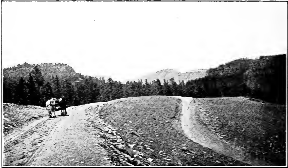
FIG. 45.—Excellent switchback layout on spur location. Note grade flattened on curve.
