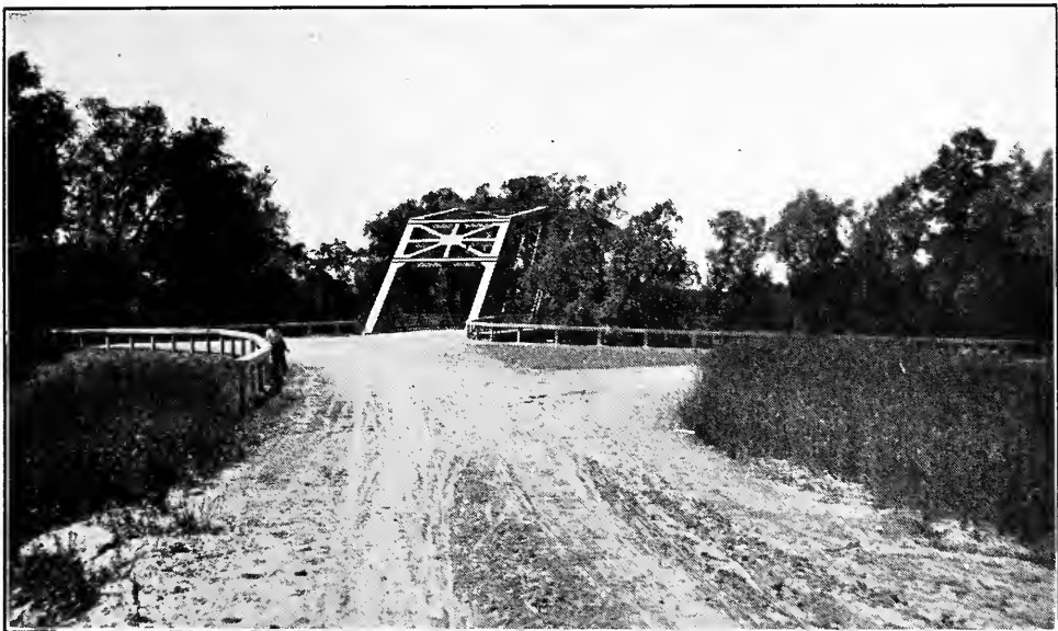
FIG. 11.—Substantial modern bridge with well designed approach protected with concrete guard rail.
