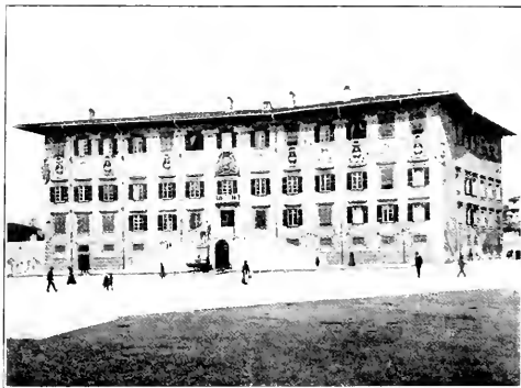
PALACE OF THE CAROVANA, PISA Rebuilt by Giorgio Vasari
