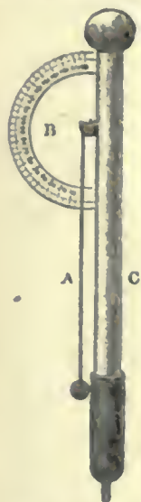
FIG. 1.—Henley's Electroscopes.
