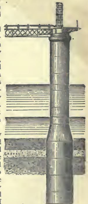
FIG. 35.—Cylinder, Charing Cross Bridge.
