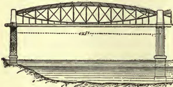
FIG. 18.—Span of Saltash Bridge.
