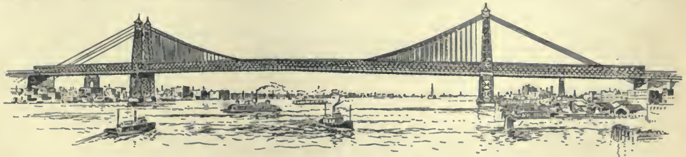
FIG. 12.—Williamsburg Bridge, New York.
