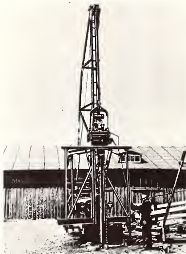
Fig. 31. The Hidroénergoproekt vibrodrilling rig mounted on an NATI tractor.
