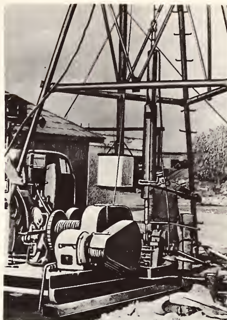
Fig. 35. Vibrodrilling rig designed by Lengidroenergoproekt, with immersible vibrator.
