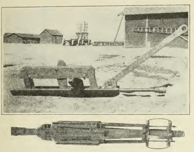
Fig. 23.—Single-blade (upper) and multiblade (lower) casing-perforating tools.
