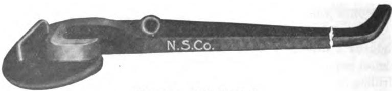
Fig. 56. Tool Wrench
