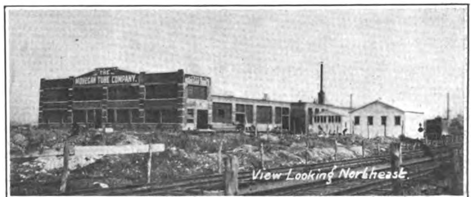
This Plant, Operated by the Mohegan Tube Company, at Scott Avenue and Meserole Street, Brooklyn, N. Y., is Busy with Orders for All Kinds of Tubing
