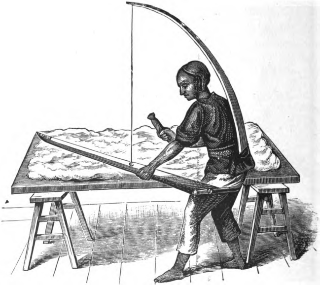
FIG. 11.—Bowling of Cotton as practised in India and China.
