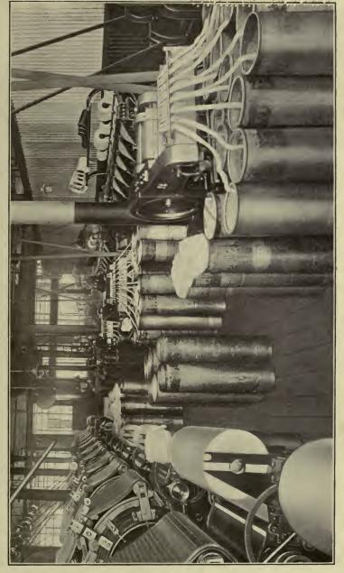
card clothing is placed upon rollers, and in the other upon a series of jointed flats which present an unbroken surface to the cotton as they revolve round the cylinder.
