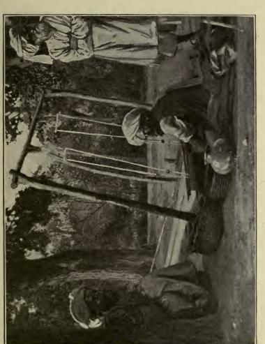
(Weaver seated in a hole dug in the ground. He works the shafts with his feet. Warps, being close to the ground, are conditioned by the moisture from the soil.) HANDLOOM WEAVING IN NORTH-WEST FRONTIER PROVINCE OF INDIA.
