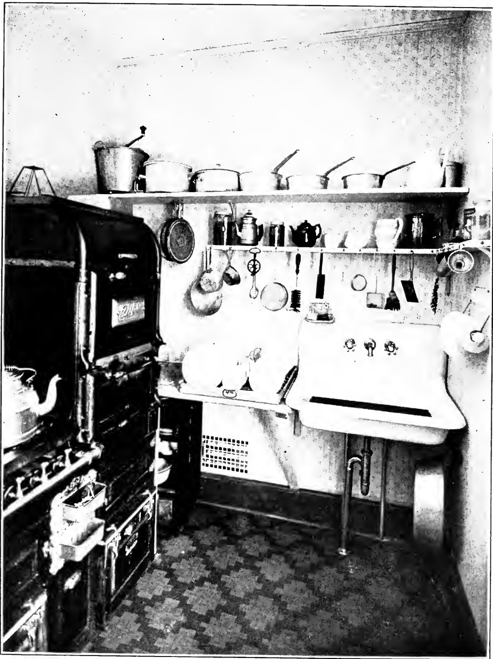
KITCHENETTE WITH GAS-RANGE.
