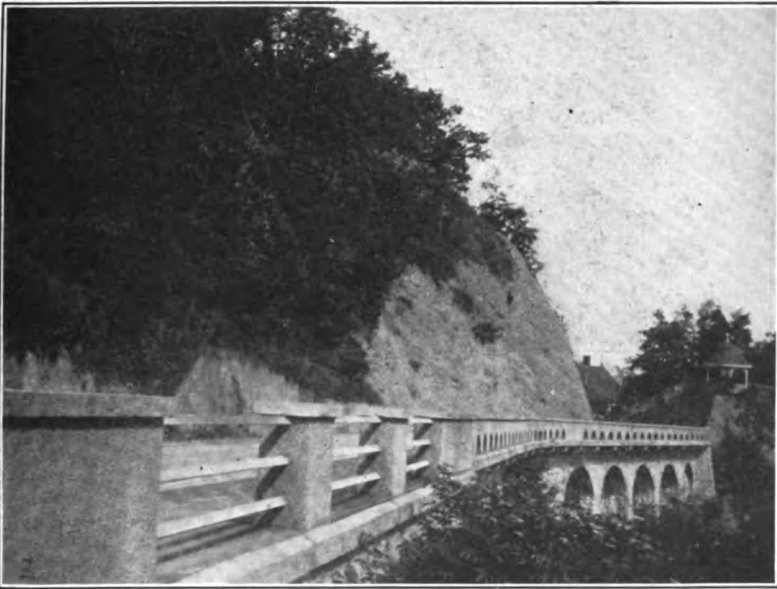
FIG. 510.—Highway structure, St. Gallen, Switzerland. (Note rough stubble finish.)
