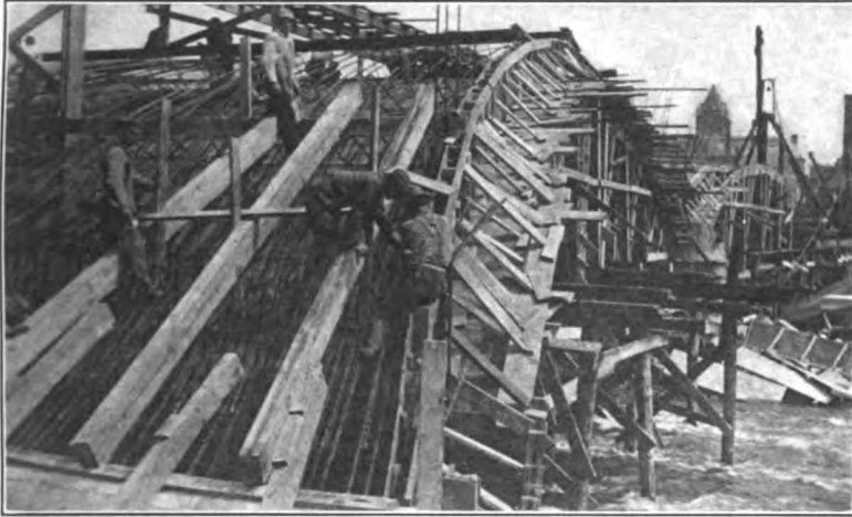
FIG. 148.—Longitudinal bulkhead used in arch-ring construction.
