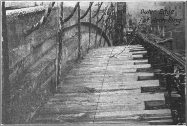
FIG. 150. —Arch ready for the building of spandrel walls.
