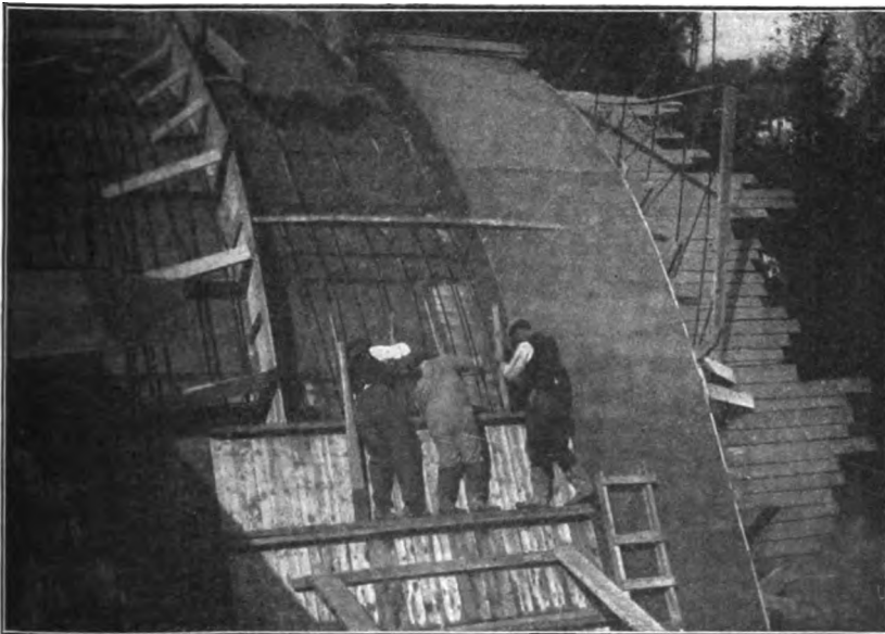
FIG. 86.—Concreting longitudinal rings, 50-ft. span, Plymouth, Mass
