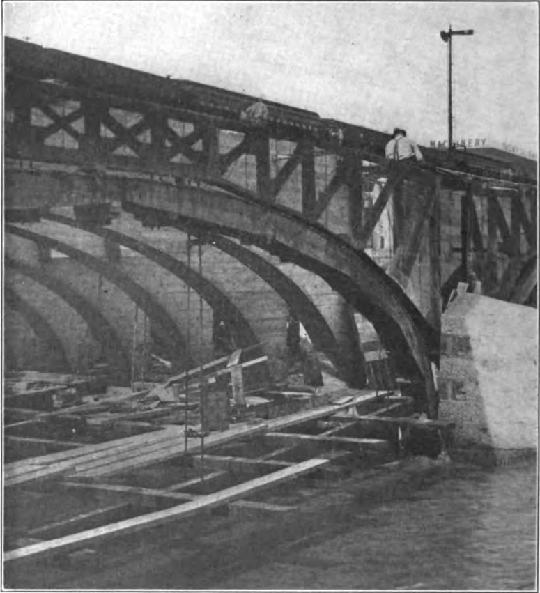
FIG. 111.—Bridge at Central Avenue, Rochester, N. Y. Structural reinforcement and arch-rib forms in place.
