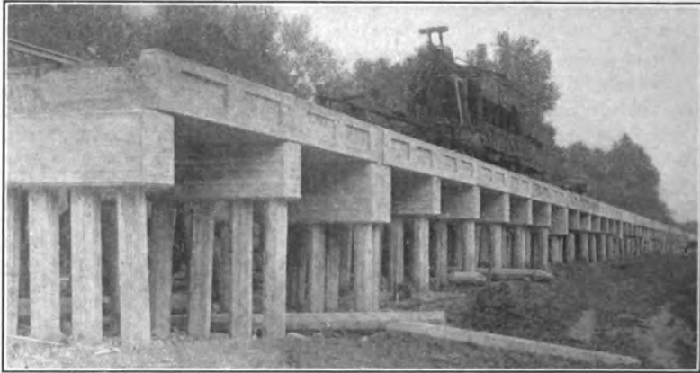
FIG. 448.—Pile trestle. General type of concrete pile trestle for crossings of more than ten spans, Illinois Central R. R. (Note the double row of piles which occurs at every sixth bent.)
