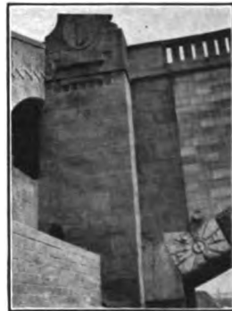
FIG. 492.—New Neckar bridge, Mannheim, Germany. (Note hinge and expansion joint through spandrel and balustrade. Also note building under arch containing apparatus for experiments.)
