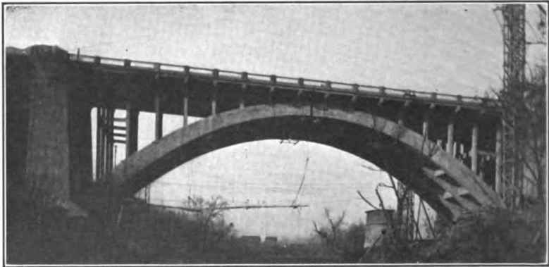
Courtesy of Mr. S. W. Bowen of Brenneke and Fay, Consulting Engineers, St. Louis. FIG. 179.—225-ft. arch span of the Main Street viaduct, Fort Worth, Texas.
