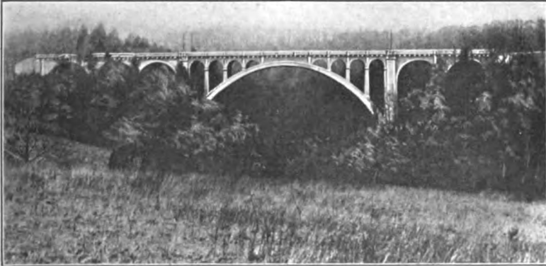
FIG. 372.—Appropriate design for great height and long span. Unfortunately the arches of the approaches do not harmonize with the spandrel arches.
