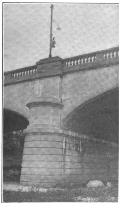
FIG. 74. —Third Street bridge, Dayton, Ohio.
