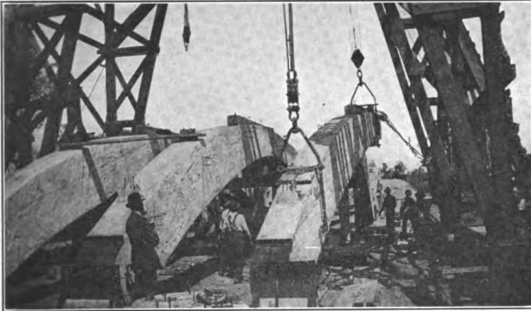
FIG. 166.—Thomas Method of arch construction.
