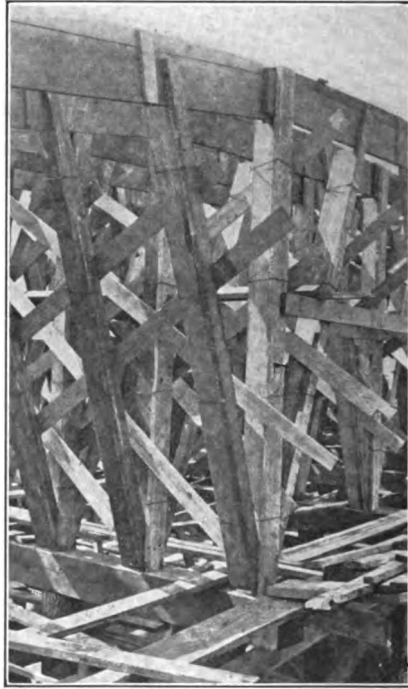
FIG. 120D.—Luten arch centering.
