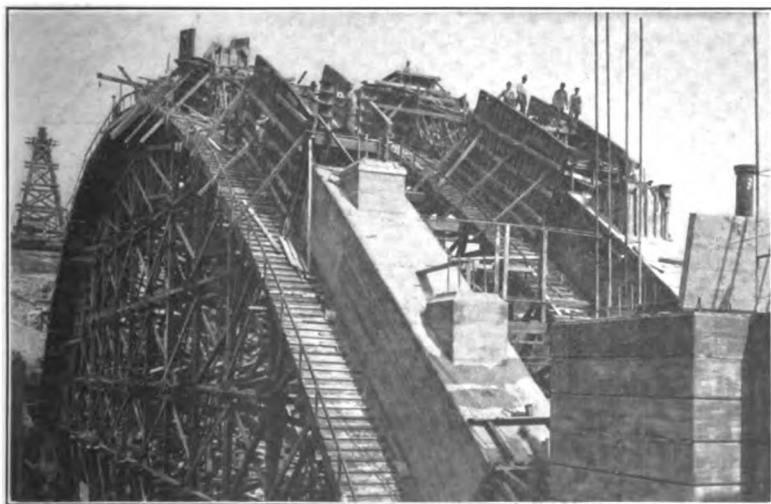
FIG. 223. —Concreting of arch ribs, Larimer Avenue bridge, Pittsburgh.
