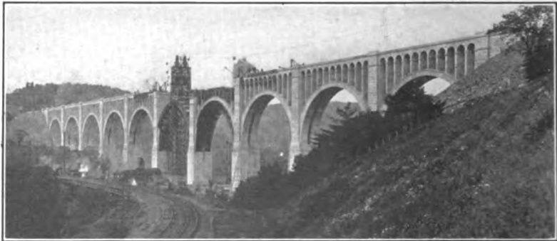
FIG. 446.—Tunkhannock viaduct. Progress photograph, June 26, 1915.
