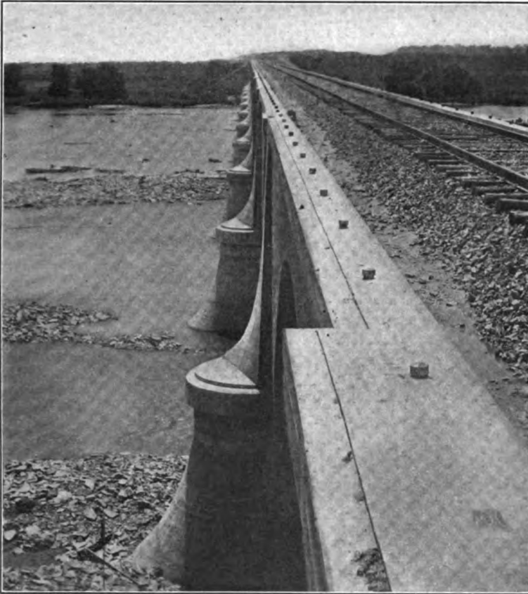
FIG. 389.—Artistic treatment of round-nosed piers, with curving batter and a triangular cutwater, blending the cocked hat of the pier cap into the spandrel face.
