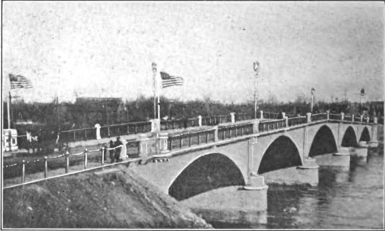
FIG. 378.—Roadway with straight grades meeting in peak at center, presenting an awkward and sagging appearance.
