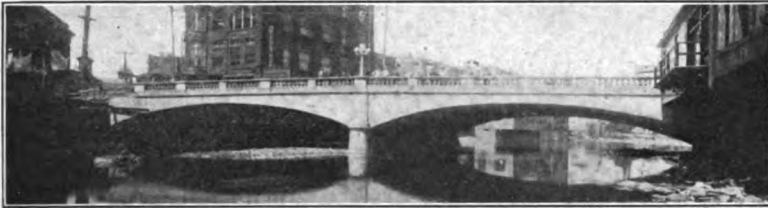
FIG. 384.—Abutments hidden, resulting in an unfortunate appearance of weakness.
