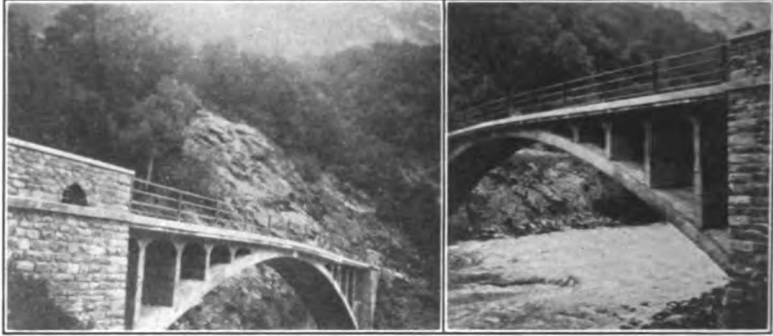
FIG. 540.—Bridge over the Glenner River near Ilanz, Switzerland.
