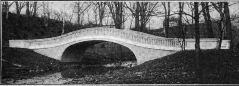
FIG. 406. —An example of Chinese camel-back design without sufficient apparent excuse. Lowering of crown would have increased the beauty of the arch curve and would have reduced the excessive reverse in the copings. Note the refuge bays at extreme ends of railing, and absence of railing detail to show end of span.
