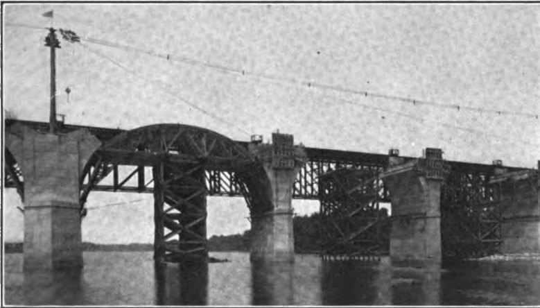
FIG. 422.—Yardley bridge. View of completed arch centering.
