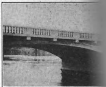
Courtesy of Engineering and Contracting FIG. 208.—Third Avenue bridge
