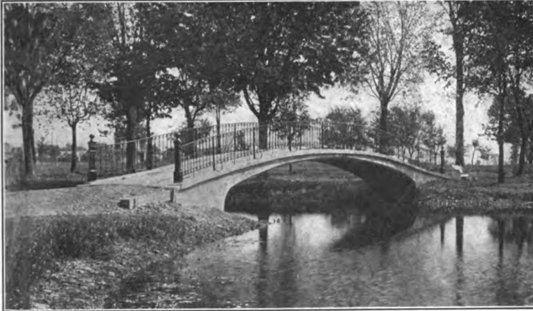
FIG. 399.—Graceful park bridge with iron railing in keeping with design. This railing would have been improved by another post over springing.
