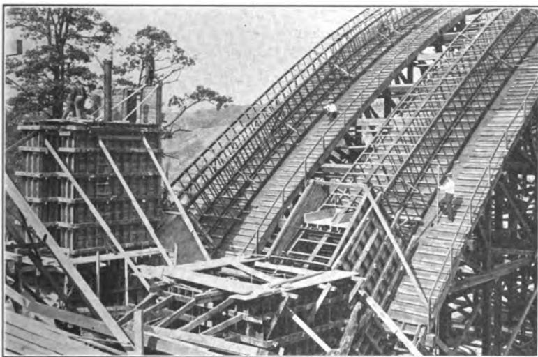
FIG. 222. —Arch-rib reinforcement in place, Larimer Avenue bridge, Pittsburgh.
