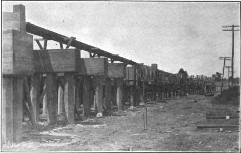
FIG. 455. —Pile trestle. Concreting pile caps from temporary narrow-gauge track carried on light framed bents.
