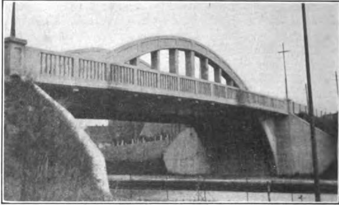
FIG. 484.—Bowstring truss over railway tracks, Friedrichsfeld, Germany.
