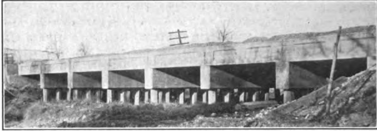
FIG. 447.—Pile trestle. General type of concrete pile trestle for crossings of less than ten spans, Illinois Central R. R.
