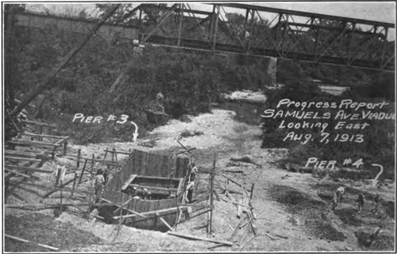
FIG. 463.—Samuels Avenue viaduct. Various stages of pier excavation.
