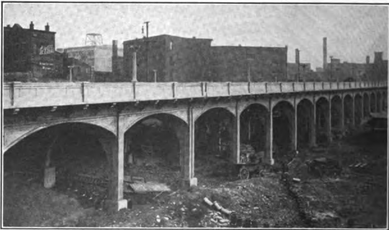
Courtesy of Mr. Frank L. Raschig, Division Engineer, Division of Structures, Cincinnati, O. FIG. 287.—Gilbert Avenue viaduct, Cincinnati, Ohio. Note expansion joint near center of illustration.
