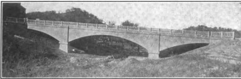
Courtesy of Mr. Frank L. Raschig, Division Engineer, Division of Structures, Cincinnati, O. FIG. 299.—Cantilever bridge on Runnymede Avenue, Cincinnati, Ohio.
