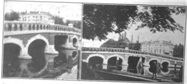
FIG. 57. Canal bridge, Rotterdam, Holland. (Combination stone, brick, and concrete.)
