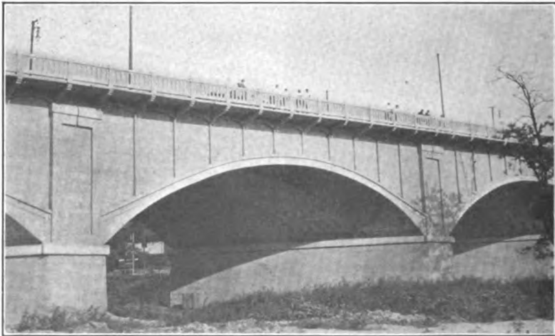
FIG. 10D.—Ludlow Avenue bridge, Cincinnati, Ohio.
