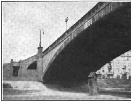
FIG. 492.—New Neckar bridge, Mannheim, Germany. (Note hinge and expansion joint through spandrel and balustrade. Also note building under arch containing apparatus for experiments.)
