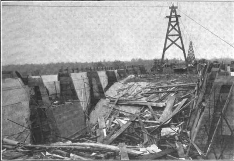
FIG. 426.—Yardley bridge. Inside view of spandrel wall forms.
