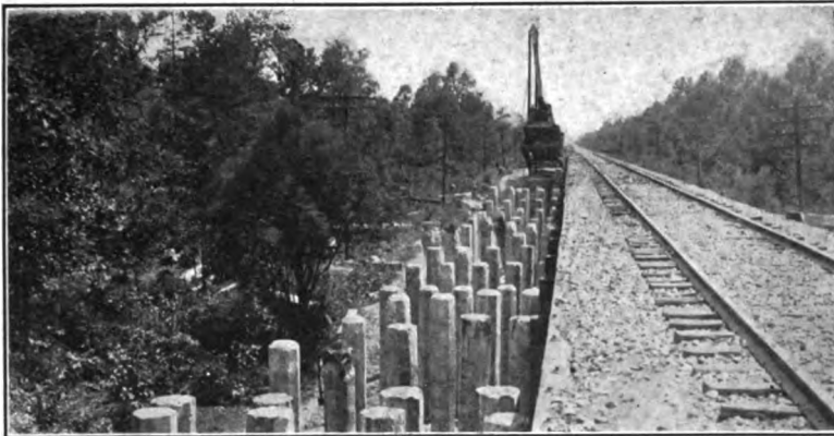
FIG. 454.—Pile trestle. Pile bents ready for pile caps. (Note excellent condition of pile heads.)
