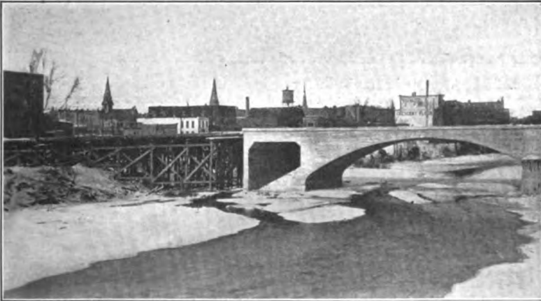
FIG. 392.—Unsightly combination of arch and box opening. Illustrates the necessity for proper treatment of abutments to show strength. The box opening is to provide for a canal which will ultimately flow along the back of a retaining wall to be erected at the abutment end of the span.
