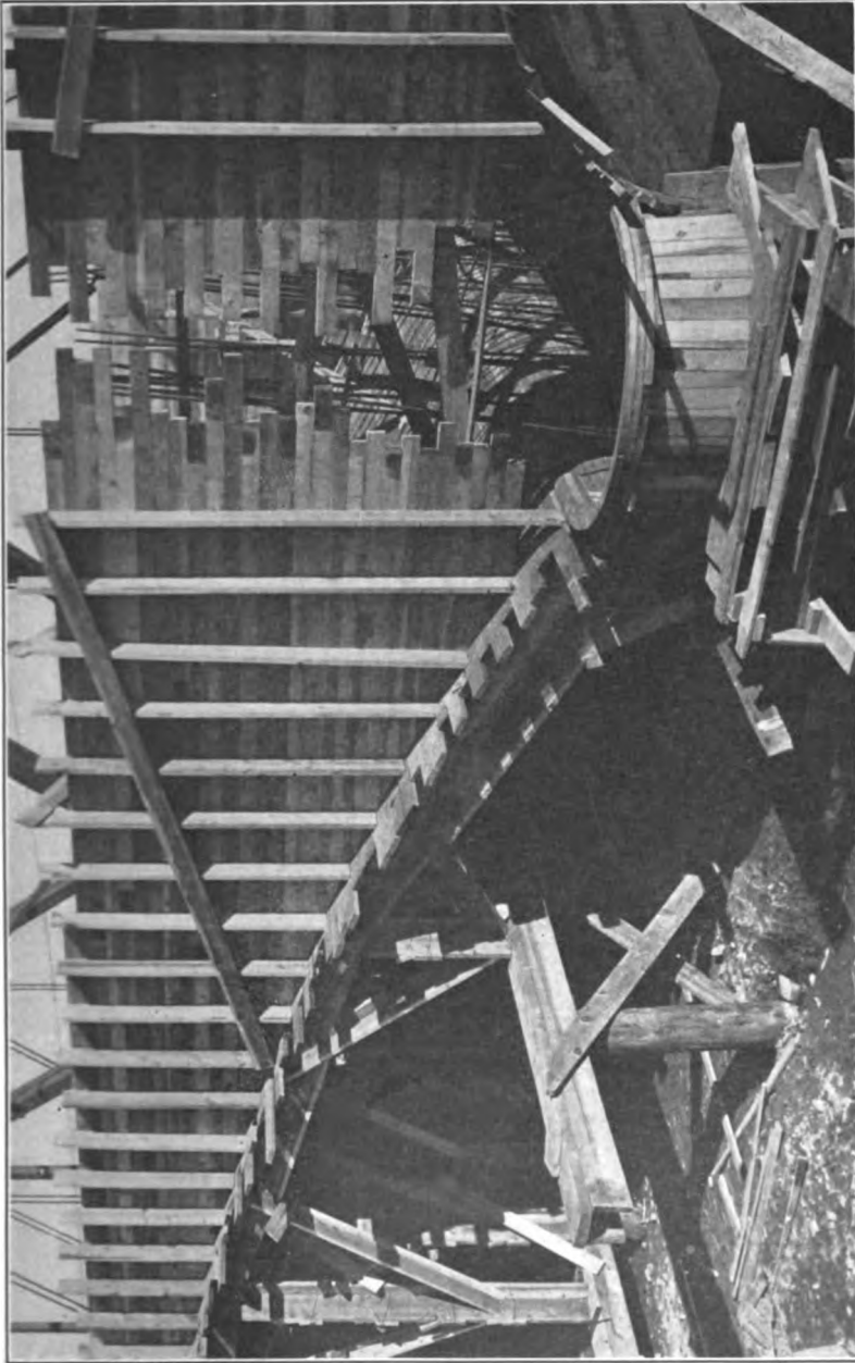
Courtesy of Mr. Daniel B. Luten, Consulting Engineer, Indianapolis. FIG. 142. —Centering and curved pier forms used in bridges of Luten Design.
