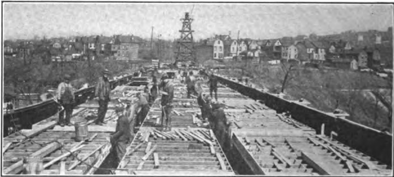
FIG. 225.—Forms for floor system over main arch, Larimer Avenue bridge, Pittsburgh.
