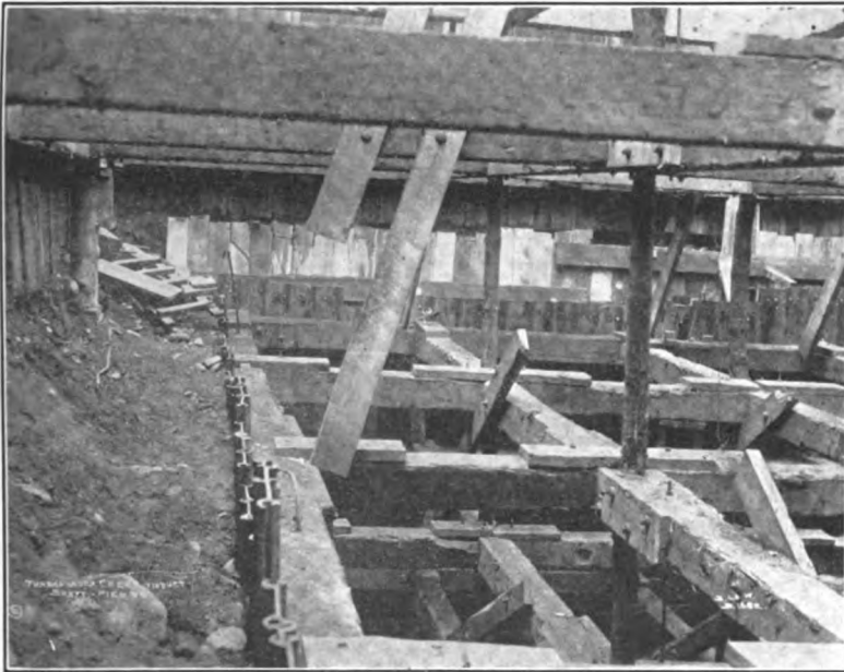
FIG. 433.—Tunkhannock viaduct. View of cofferdam at junction of outer and inner sheetings, lower ends of outer sheeting visible.
