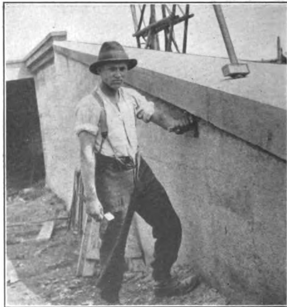
FIG. 541.—Process of surface finishing and tools required. (Note direction of tool for vertical scoriation under coping.)
