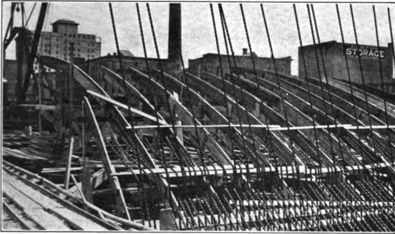
FIG. 120B.—Luten arch centering.
