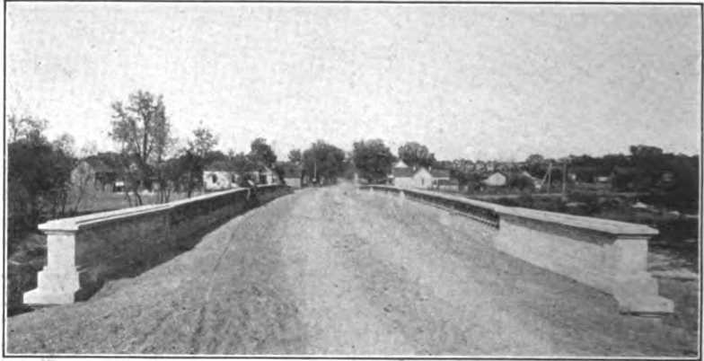
FIG. 401.—A well-proportioned railing on a three-span arch bridge. Note spandrel coping, plinth, dado, cap, solid dado over abutments and pier, true line and camber of handrail uninterrupted by posts except at abutment and piers.
