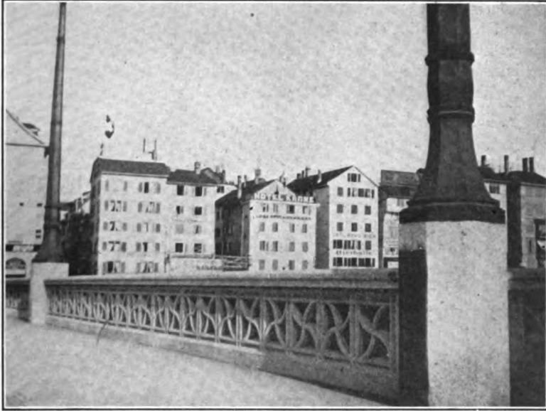
FIG. 507.—Detail view of entrance balustrade and standards, Urania bridge at Zurich. Note surface finish.
