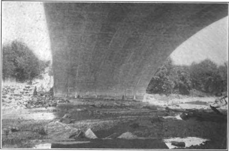
FIG. 81.—Harford Avenue bridge over Hering Run, Baltimore, Md. Showing method of construction of arch ring in longitudinal sections.
