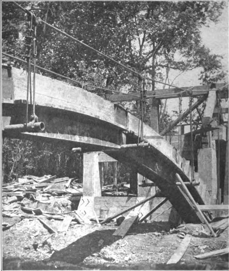
FIG. 131.—View of Chickahominy River bridge during construction. One rib completed and suspended centering ready to be removed.
