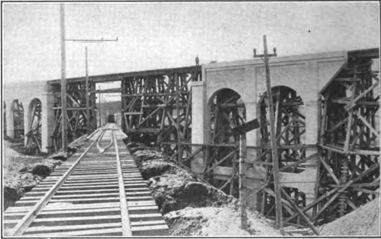
FIG. 310.—Skeleton abutments for steel truss span on Chicago, Milwaukee & St. Paul Ry. Timber trestle within abutments being removed.
