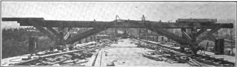
FIG. 226.—View of traveler for suspending working scaffolds for bushhammer work, Larimer Avenue bridge, Pittsburgh.
