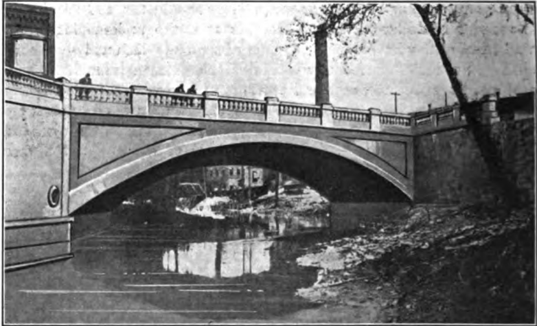
FIG. 404.—A substantial and expensive structure, yet unsightly. Arch curve awkward and improperly selected for the earth fill; excessively heavy crown; the whole effect being of constricted waterway for which there is no necessity. Objectionable railing post over crown. Drainage discharge should have been through arch instead of wing.
