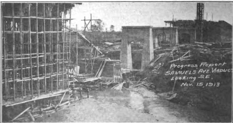
FIG. 474.—Samuels Avenue viaduct. View of river span falsework, showing also the difference in construction of river and land piers.
