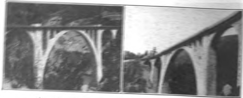
FIG. 56. Stone arches (left) and stone bridge (right).
