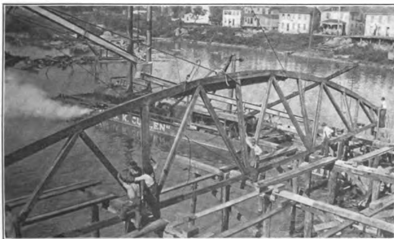
FIG. 124B.—Centering for High Street bridge, Hamilton, Ohio.
