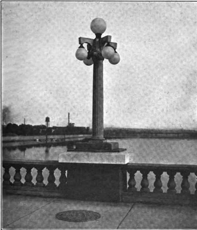
FIG. 407. —Detail of lamp post from bridge shown in Fig. 366. The post is made entirely of concrete including the brackets, with bronze holders for the glass globes. Cap of railing post is excessively heavy, but is necessitated for proper appearance of pier from water front.
