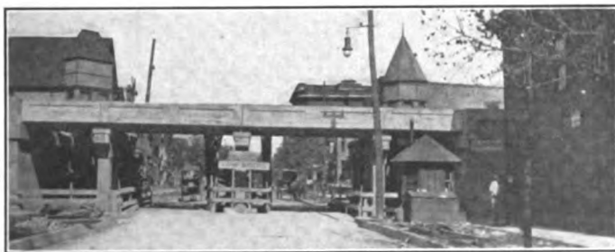
FIG. 458.—Track-elevation subways. View of 60-ft. subway, Bloomingdale Road track elevation, Chicago, C. M. & St. P. Ry.
