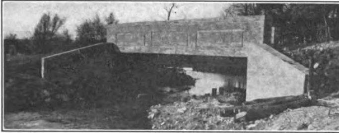
Courtesy of Mr. M. W. Torkelson, Bridge Engineer, Wisconsin Highway Commission.
