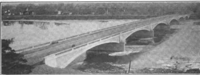
FIG. 373.—Oval arches approximating ellipses, with solid earth-filled spandrels, suitable for locations subject to floods.
