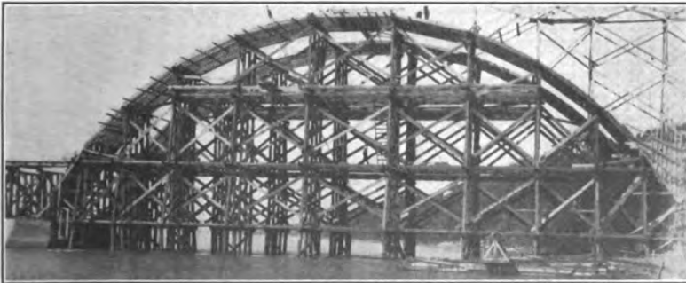
Courtesy of Mr. Daniel B. Luten, Consulting Engineer, Indianapolis. FIG. 102.—Timber falsework and centering for arches. Bridge over Saskatchewan River at Saskatoon, Canada.
