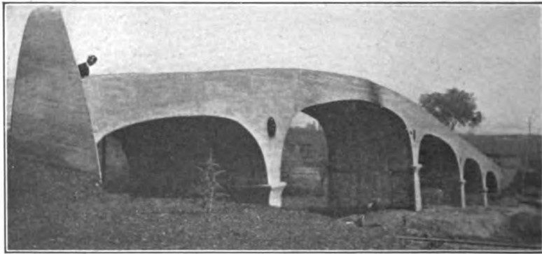
FIG. 394.—Inartistic attempt to treat concrete as an individual material; a proper motive, but handled with no knowledge of structural ornamentation. Note absence of coping, railing, pilasters, and improper attempt at ornamentation over piers.
