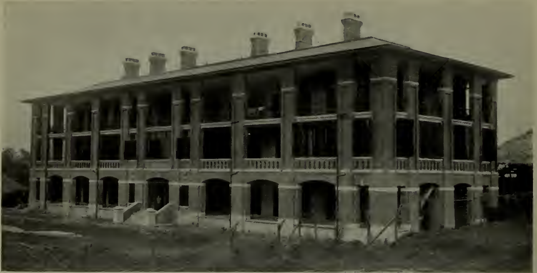
Stoughton & Stoughton, Architects. East Hall, Canton Christian College, Canton, China. Built Kahn System Reinforced Concrete.
