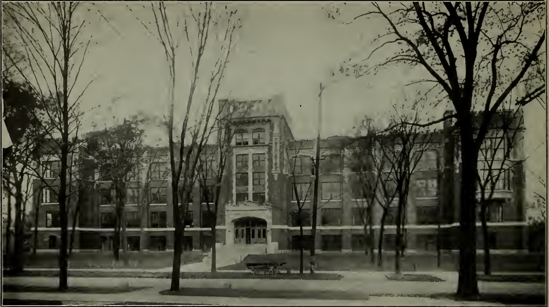
Central High School, Grand Rapids, Mich. Kahn System Reinforced Concrete Used Throughout.
