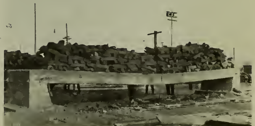
Deflection of 6 in. before Gradual Failure at Center Under Load of 52,000 lbs. (375 lbs. per sq. ft.) Five times the designed load.
