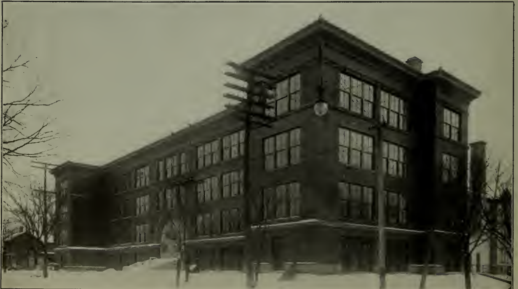
Union High School, Grand Rapids, Mich. Kahn System Reinforced Concrete Used Throughout.
