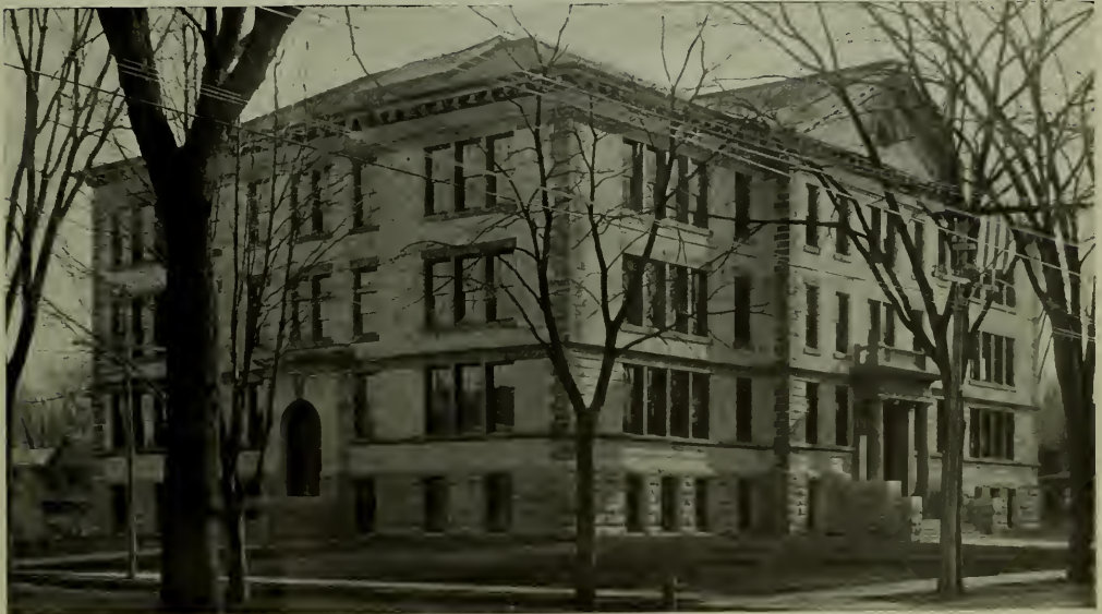
Union High School, Glens Falls, N. Y. Kahn System Reinforced Hollow Tile Construction Used Throughout.
