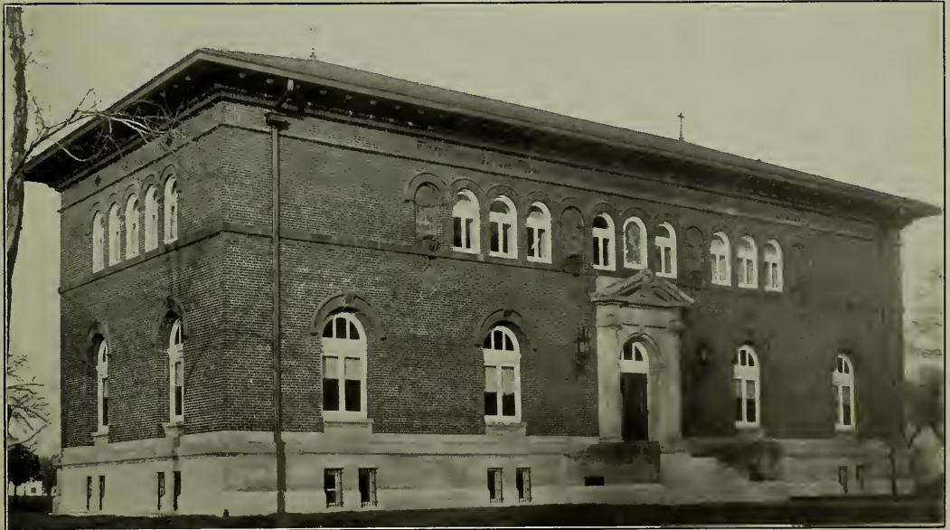
Art Building, St. Marys of the Springs Academy, Columbus, Ohio. Built Kahn System Reinforced Concrete.
