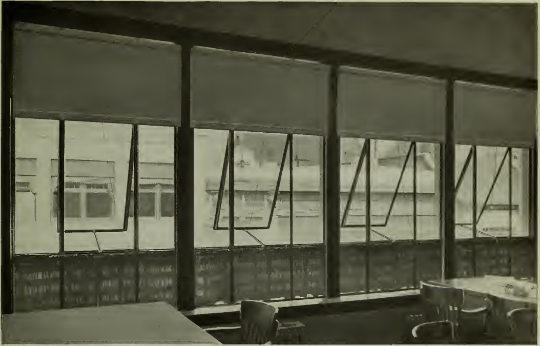
Economy Casements of United Steel Sash. A Type Well Adapted to School Buildings.
