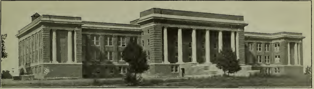
Main Building, Tennessee State Normal School, Memphis, Tenn. Kahn System Reinforced Concrete Used Throughout.
