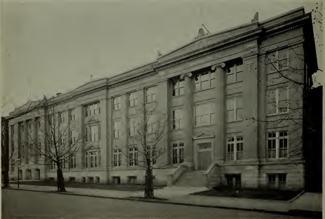
Frank G. Pierson, Architect. Gonzago College, Washington, D. C. Floors of 37 ft. Span, built Kahn System Reinforced Concrete.
