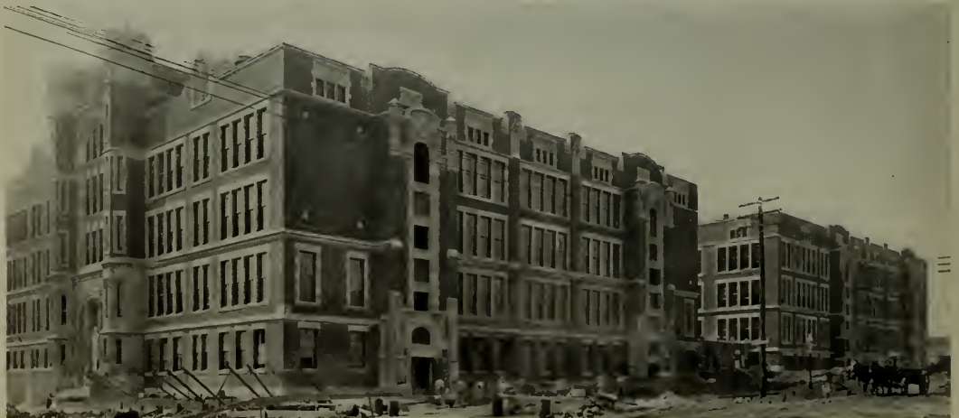
West Philadelphia High School, Philadelphia, Pa. Kahn System Reinforced Concrete Used Throughout.
