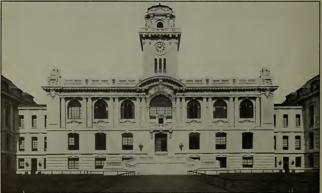
Buildings for U. S. Naval Academy, Annapolis, Md. Ten Kahn System Buildings in this Group.
