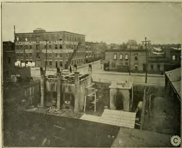
The entire building was constructed of concrete and provided with six chimneys and eight draft openings at the bottom, with two openings closed by doors for putting in the fuel.
