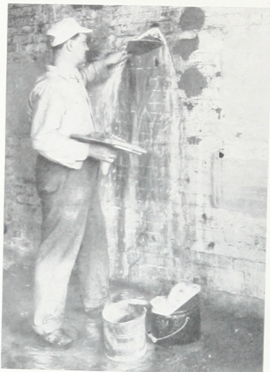
Repair cracks and holes against water pressure
