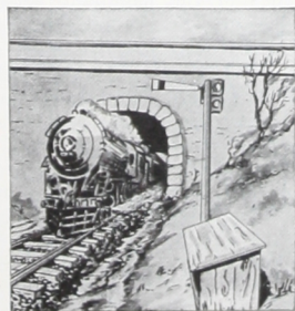
Railroad tunnels are leak-proofed and plaster-coated with FLEXTITE
