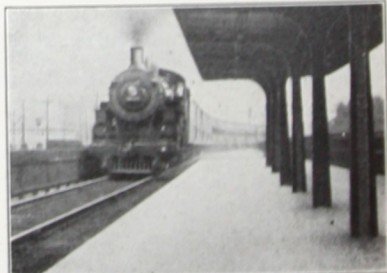
Repair and resurface Station Platforms with RUGGEDWEAR RESURFACER
