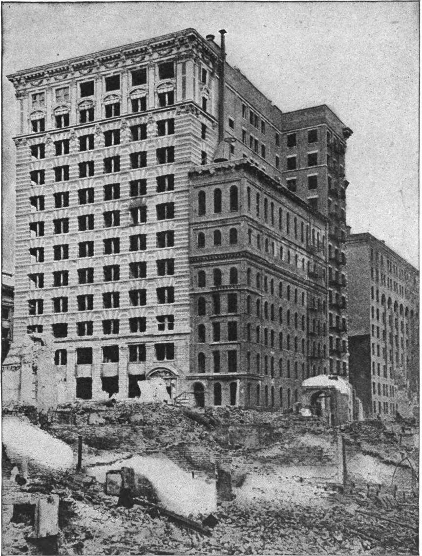
Fig. 13. One of the Big Brick and Terra Cotta Baltimore Buildings after the Fire The contents gutted but the exterior nearly intact.
