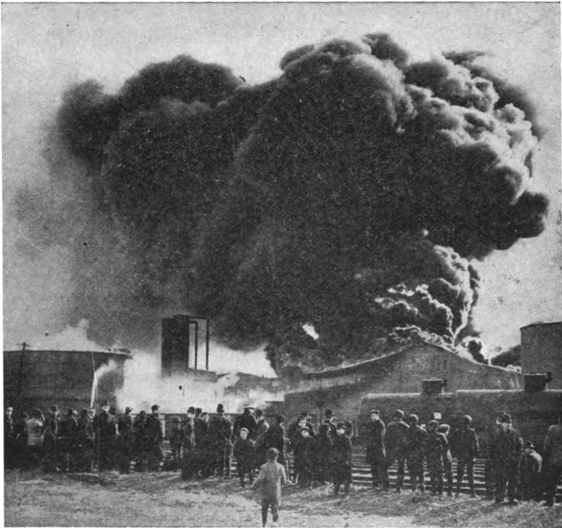
Fig. 50. Standard Oil Tanks Ablaze—A Dangerous Risk to Handle
