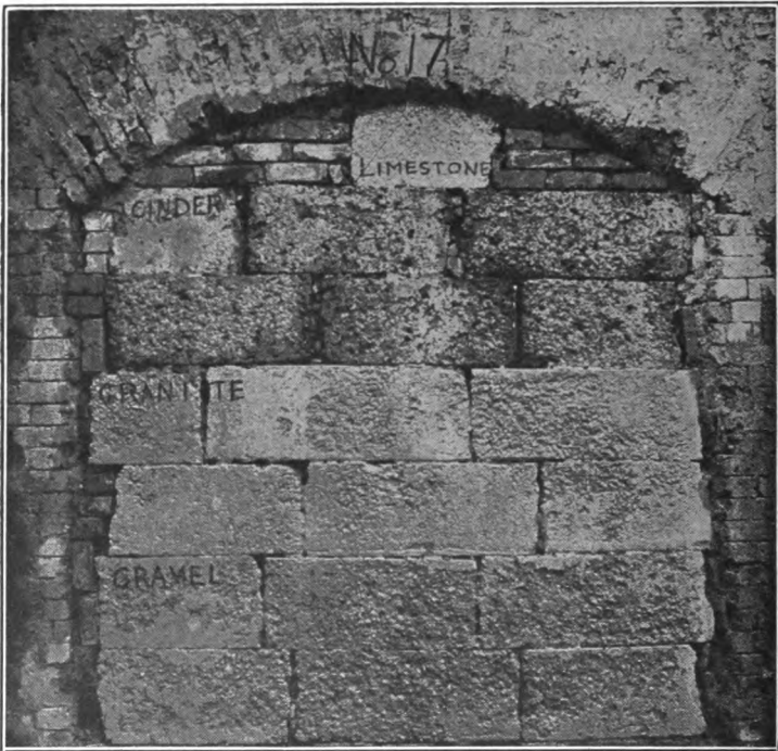
Fig. 114. Appearance after Test of Panel Consisting of Different Kinds of Concrete
