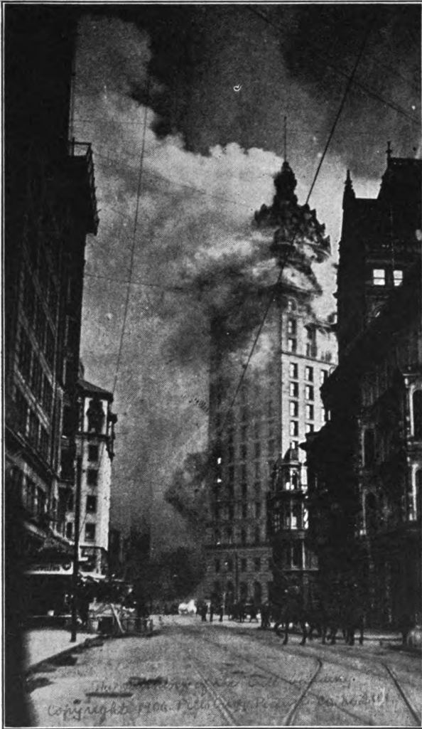
Fig. 26. Fire's Ingress via the Window Route
