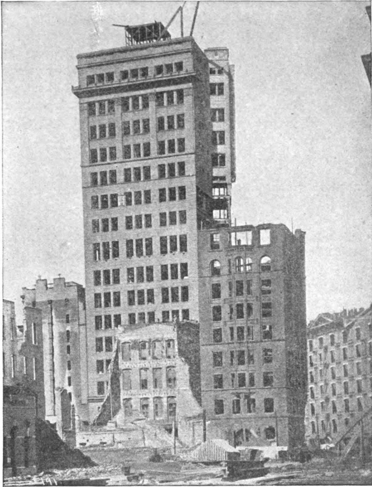
Fig. 10. The Almost Completed Chronicle Building in the San Francisco Fire Nothing in it to burn but a little scaffolding so that it was virtually uninjured
