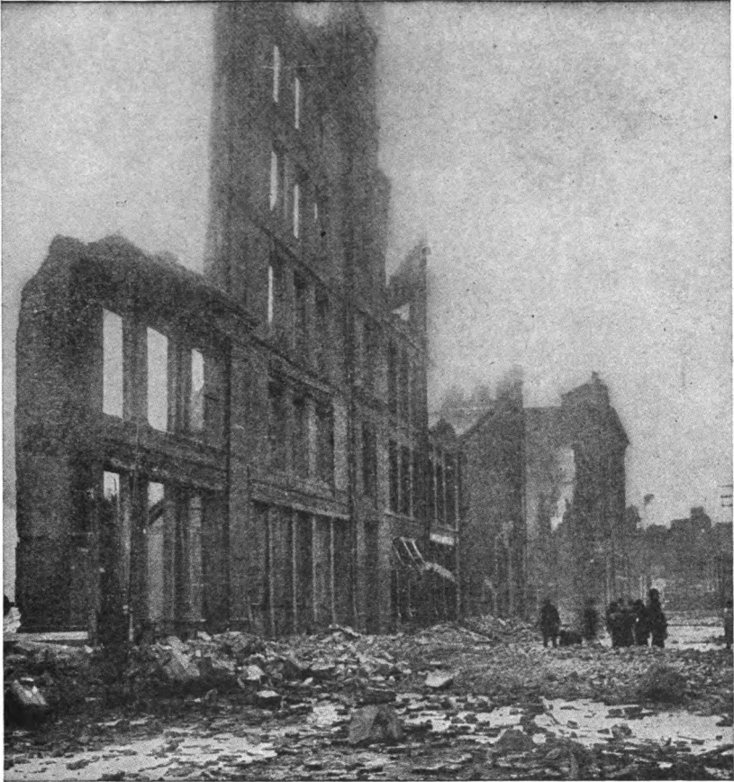
Fig. 8. The Hurst Building where the Baltimore Fire Started
