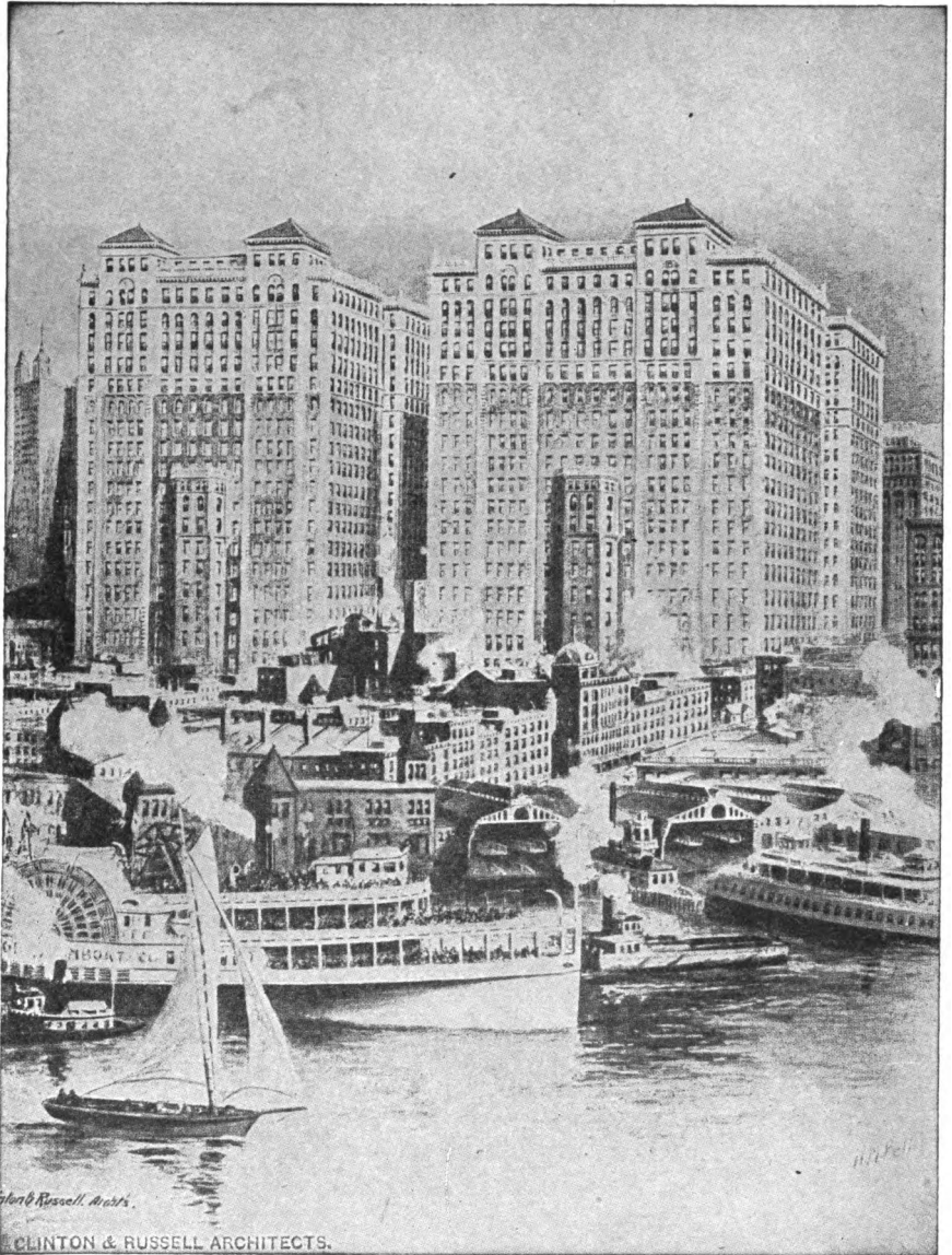
Fig. 19. The Largest Office Building in the World—The Hudson Terminal, New York City Well fireproofed but a bad exposure in that it is surrounded by a miserable lot of fire-traps
