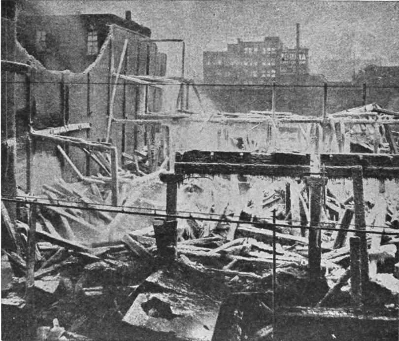
Fig. 28. Another "Slow-Burning" Fire; 33 Minutes Destroyed the Usefulness of This Building
