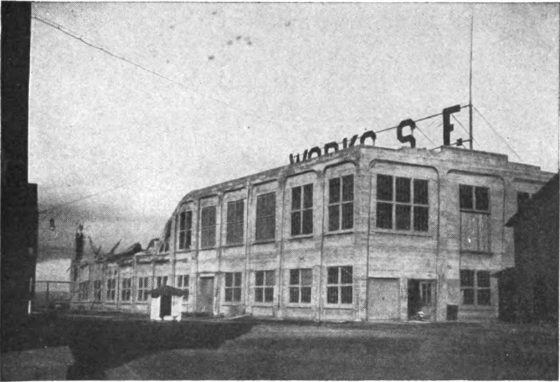
Fig. 107. Effects of a Fire in the Rubber Reclaiming Manufacturing Plant
