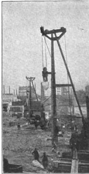
Fig. 52.—View of Apparatus Used in Constructing Compressol Piles.
