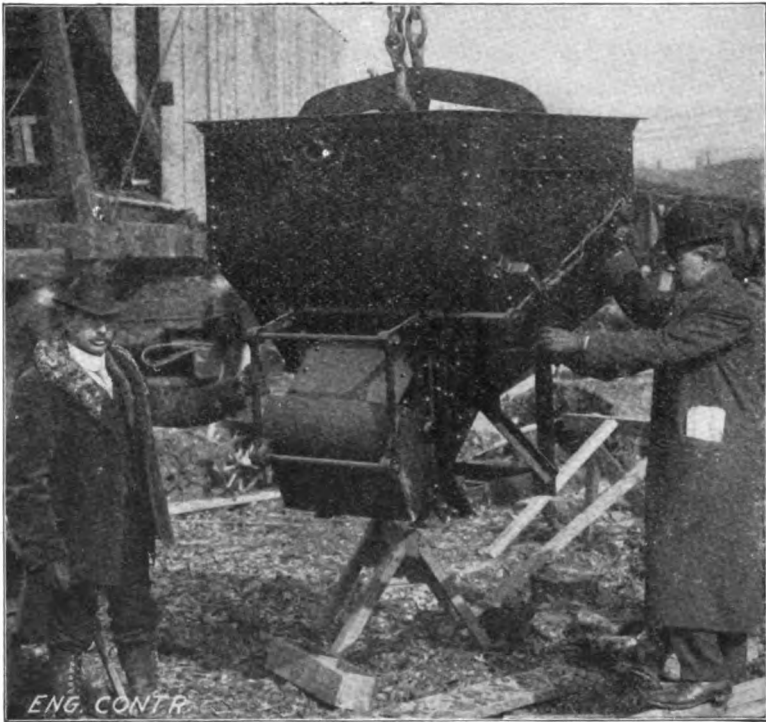
Fig. 222.—Special Concrete Bucket for Large Warehouse Building.
