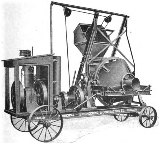
Fig. 19.—Chicago Improved Cube Concrete Mixer with Elevating Charging Hopper.
