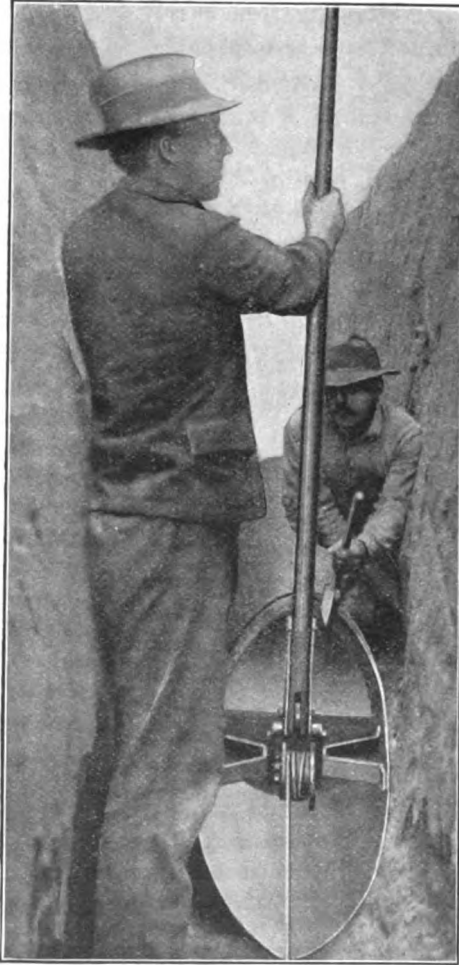
Fig. 268. —Ransome Continuous Mold for Concrete Pipe Construction.
