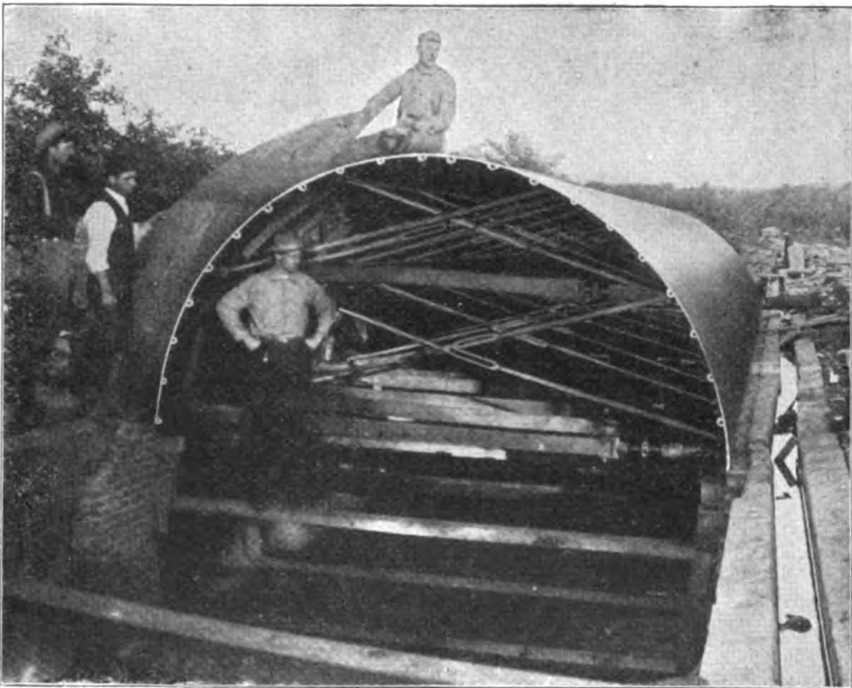
Fig. 247. —Blaw Collapsible Steel Centering for Conduit Construction.
