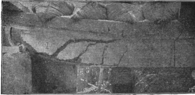
FIG. 134.—Beam I, cracks in the end without stirrups at the breaking load.
