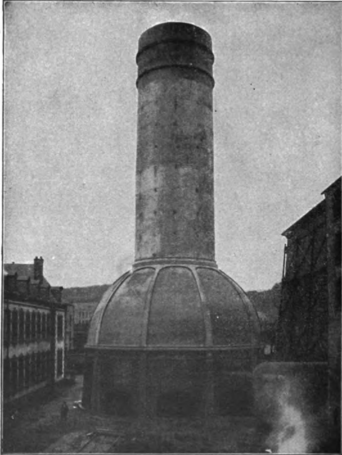
FIG. 346.—Cooling tower of the Differdingen Steel Works.
