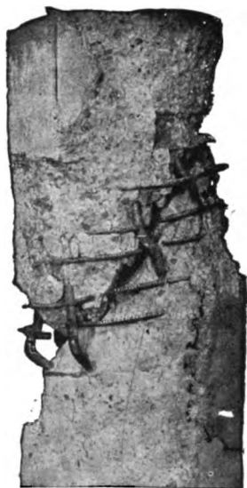
FIG. 72.—Failure from shear. (Spiral broken.)
