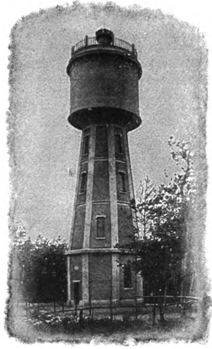
FIG. 316.—Water tower in Rixensart.
