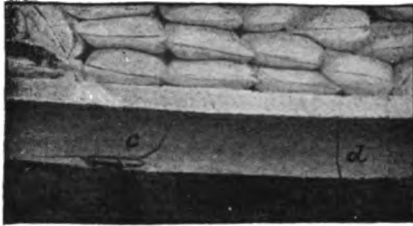
FIG. 170.—Bursting effect of loose diagonal stirrups.
