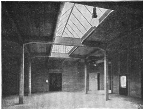
FIG. 230—Krefeld warehouse, with flat roof and monitor skylights.
