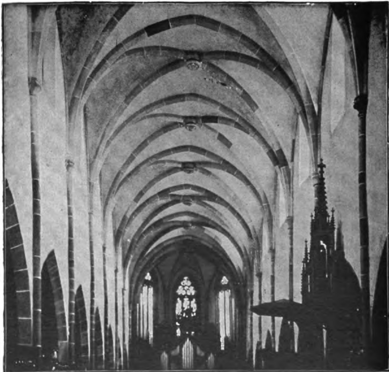
FIG. 245.—Groined arches of reinforced concrete in the monastery chapel in Landau.
