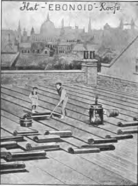
LAYING AN "EBONOID" ROOF IN LONDON.
