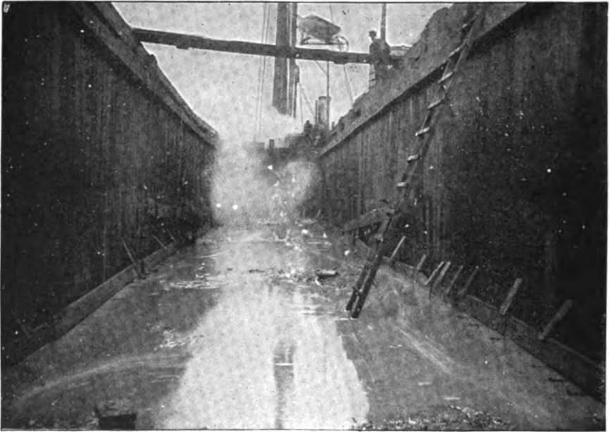
FIG. 86.—COFFER-DAM ON CHARLESTOWN BRIDGE.
