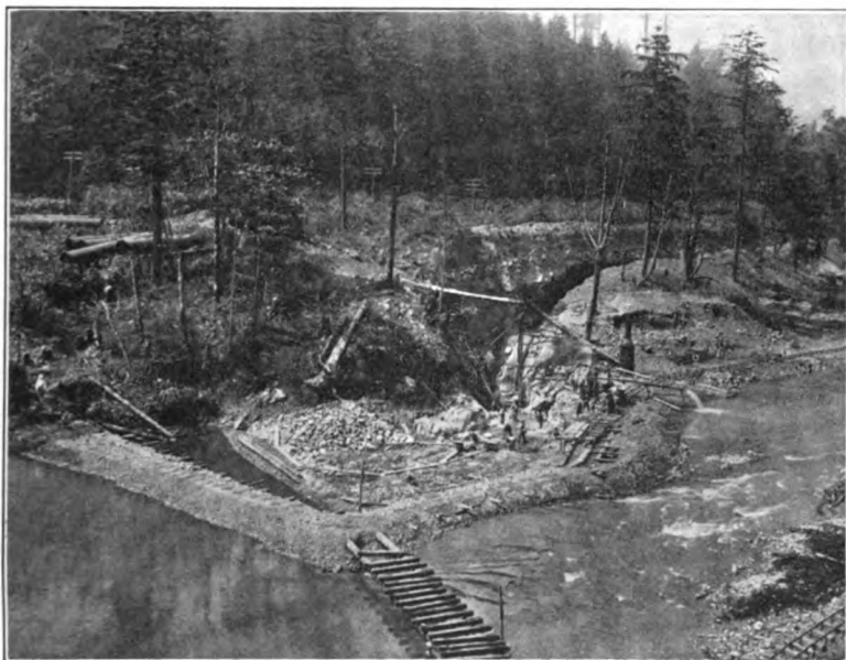
FIG. 21.—GREEN RIVER LOG CRIB COFFER-DAM.
