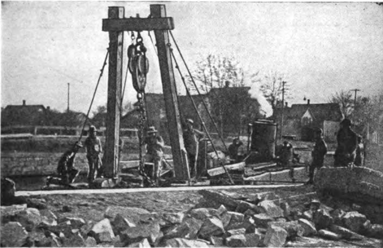
FIG. 51.—PILE-PULLING SCOW, NEW YORK STATE CANALS.
