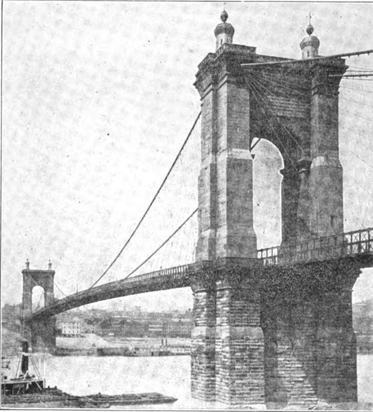
FIG. 162.—CINCINNATI SUSPENSION BRIDGE.
