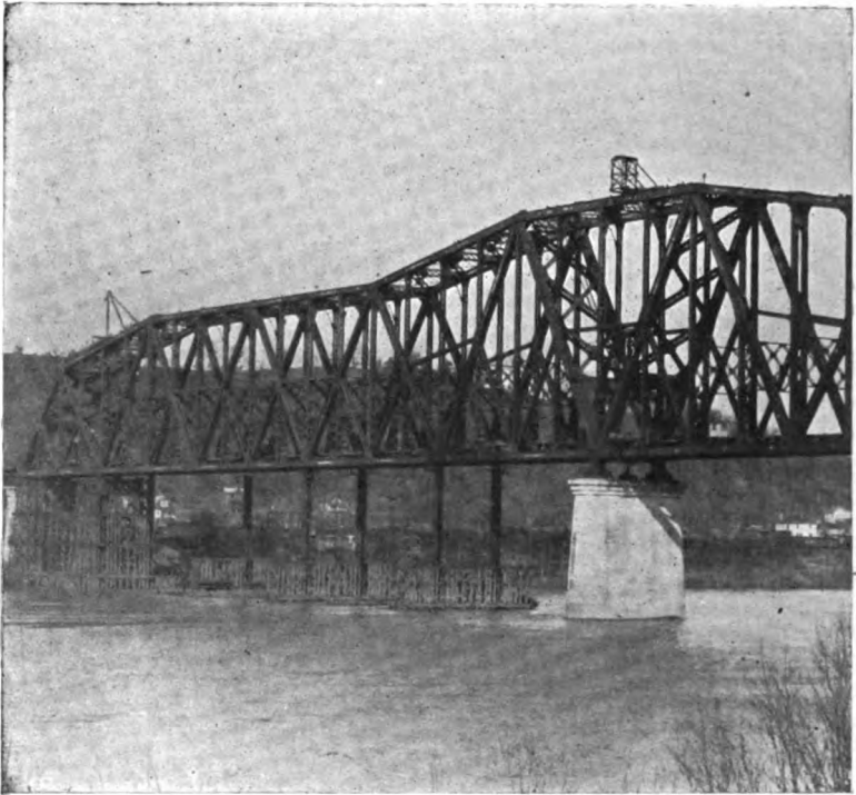
FIG. 252.—CHANNEL PIER, SCIOTOVILLE BRIDGE.
