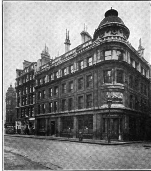
VIEW ALONG EASTCHEAP, SHOWING PEEK HOUSE
