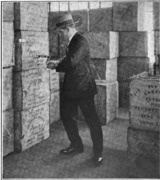
Boring sample hole with special auger.
