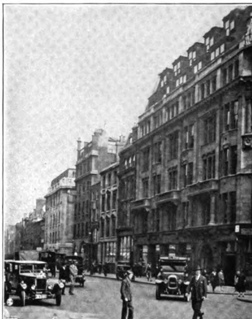
A VIEW IN GREAT TOWER STREET Harrisons & Crosfield building on the right.
