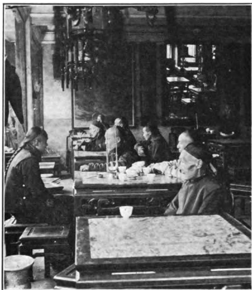
TEA-HOUSE INTERIOR, SHANGHAI
