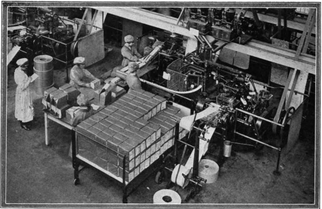
ONE OF THE AUTOMATIC PACKETING MACHINES WITH OVERHEAD ELECTRIC WEIGHERS
