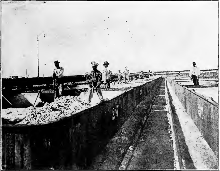
FIG. 49.—Deposit of nitrate crystals in the pans of Fig. 48 after the liquor is run off.
