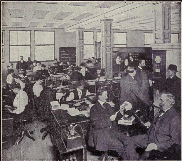
VIEW IN GENERAL OFFICE
