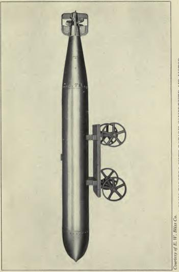
A BLISS TORPEDO WITH ROTARY COMPRESSED AIR MOTOR
