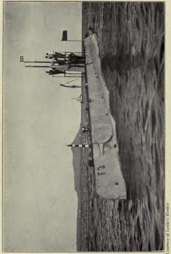
A MODERN AMERICAN SUBMARINE CRUISING IN THE AFLOAT CONDITION WITH FOREWARD DIVING. RUDDERS FOLDED BACK AGAINST THE HULL
