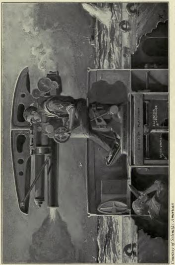
A 3<sup>15</sup> INCH SUBMARINE GUN IN ACTION SHOWING THE DECK WELL AND MANNER OF OPERATION
