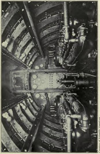
Courtesy of Scientific American THE ENGINE ROOM OF A MODERN SUBMARINE SHOWING THE DIESEL ENGINES
