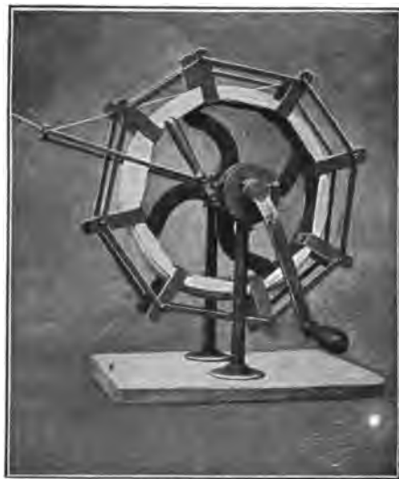
Old Pulleys and Pipe Fittings
