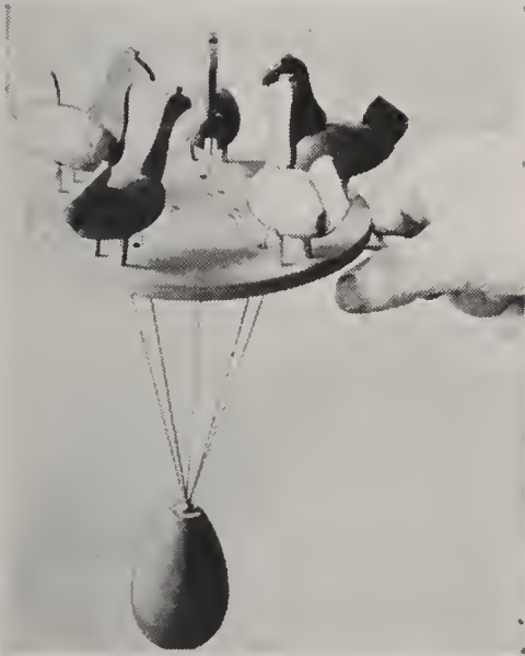
FIG. 653.—THE FEEDING-HENS TOY IS WORKED BY A PENDULUM. (See Chapter XLII.)
