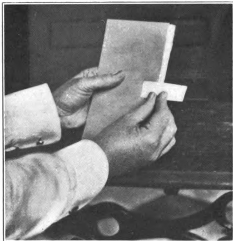
PLATE XLVII. Determining the distance between covers.
