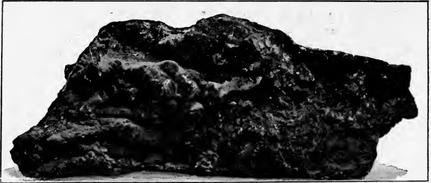
EXHIBIT NO. 3. SCALE BETWEEN THE TUBES NEAR BOTTOM OF BOILER, CAUSING TUBE TO LEAK. (John Wanamaker, 1825-1829 Market St., Philadelphia, Pa.) Water used—Schuylkill River water.
