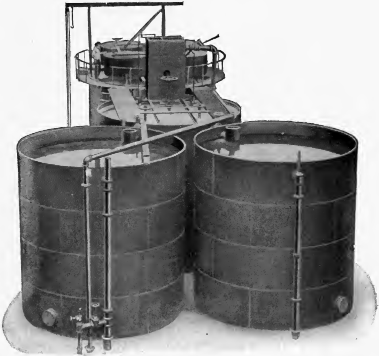
FIG. 49.—Water-softening Plant of Proctor and Gamble Co., Ivorydale, Ohio.
