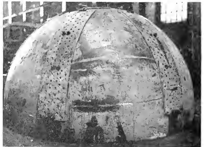
Fig. 3.—Head in Process of Assembly
