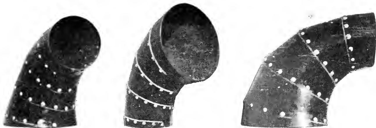
Three Views of the Spiral Sheet Layout of a Transition Elbow
