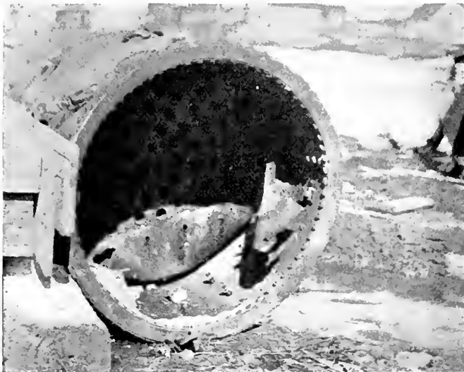
Fig. 1.—Shell of Boiler After the Explosion
