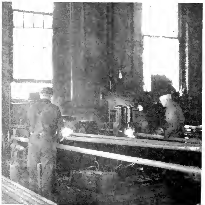
Fig. 9.—Welding Furnaces and Pneumatic Welders in Action
