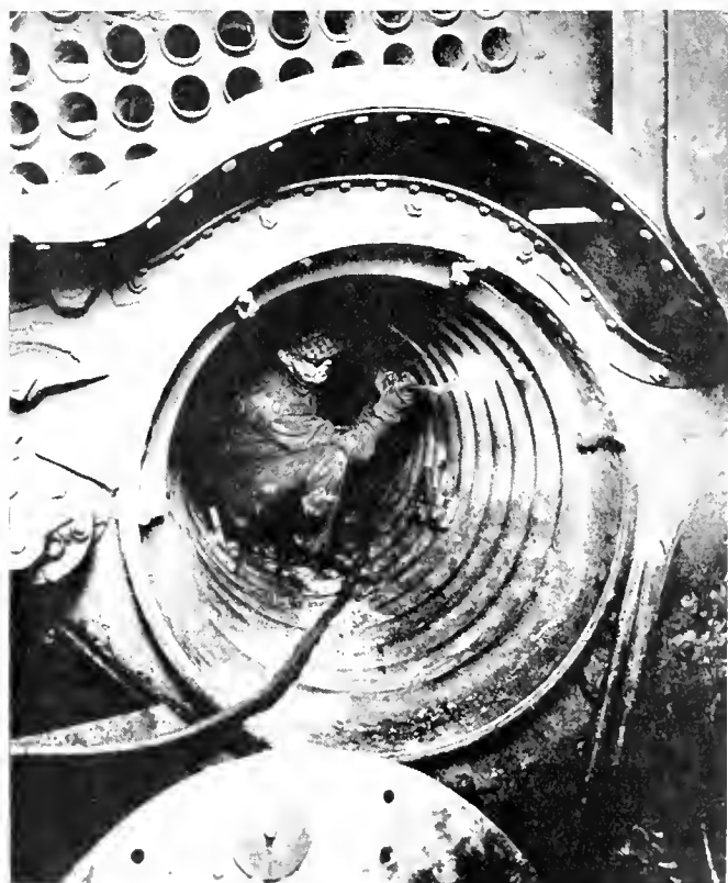
Fig 2.—Cutting out Burned Section of Scotch Marine Boiler Furnace
