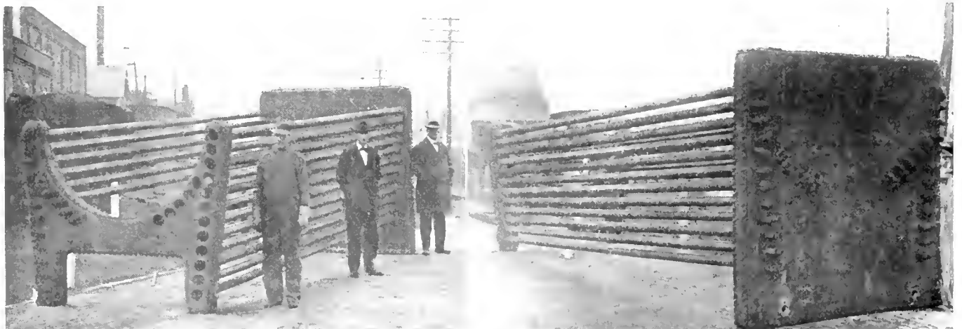
Two Types of Water Tube Economizers for Horizontal Return Tubular Boilers
