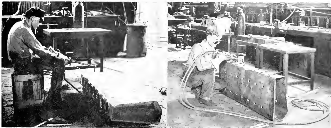
Fig. 1.—Welding Operations on Smoke Consumer
