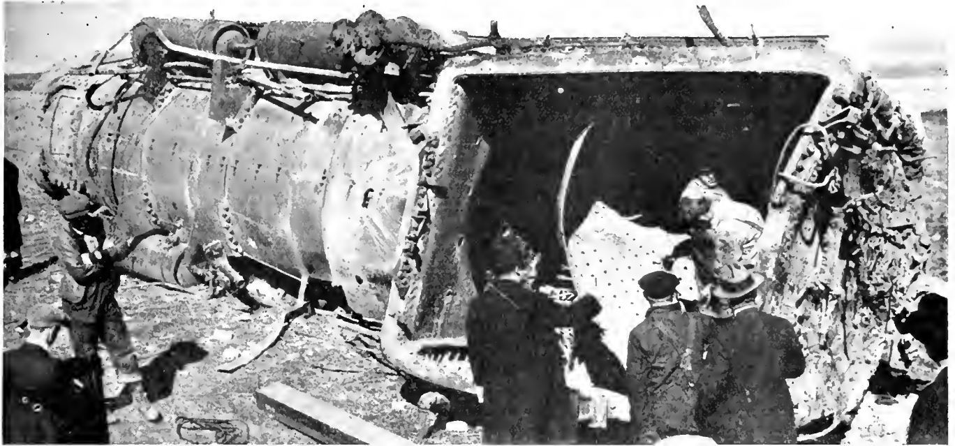
Firebox Wreckage after Great Northern Locomotive Low Water Explosion
