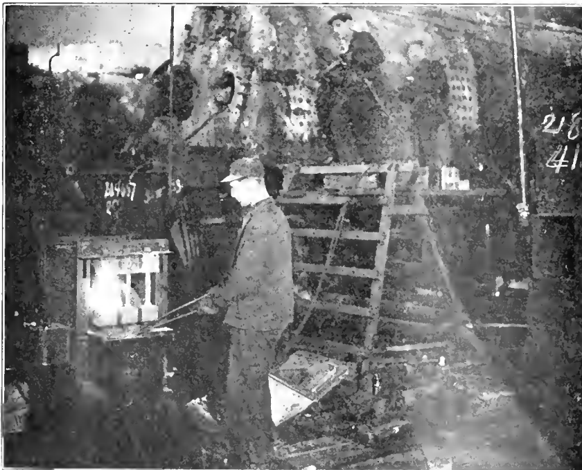
Calorac 3-Head Portable Rivet Heater on Boiler Work
