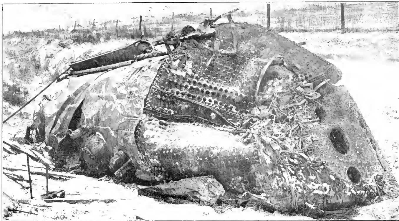
Fig. 2.—Wreck of Boiler Which Landed About 350 Feet from Point of Accident
