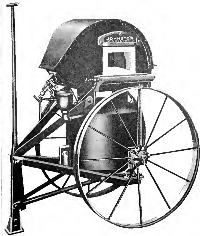
New Oil Burning Rivet Forge
