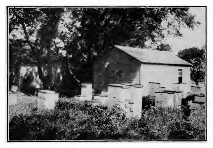
Fig. 54. Honey-house built so that it may be readily cut apart into sections and removed. Where the cut is to be made, rafters or studding are placed within an inch of each other and holes bored so that the sections may be drawn together with bolts when set up again.
