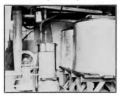
Fig. 61. Settling tanks and heating system are in the basement of the Sutton central plant.
