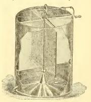
tracts from four combs at once, but also reverses or changes sides with the combs after one side has been extracted thus presenting the other side simply by reversing the motion of the crank.
