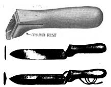
Fig. 121—Bingham Uncapping-Knife. Fig. 122—Steam-heated Uncapping Knife.
