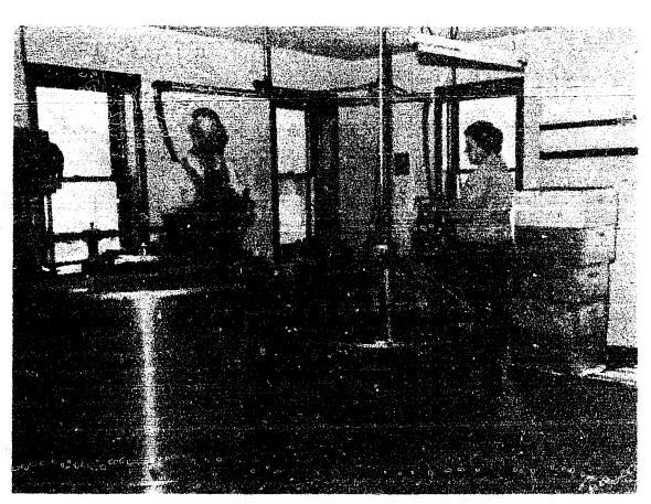
Neatness and efficiency makes working in the honey house a pleasure. Note the merry-geround for uncapped combs placed between the uncapper and the extractor.
