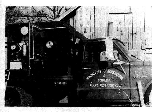
Truck-mounted furnigator used in Virginia. Centrol box showing gauges which indicate temperature and pressure, the measuring flask on hanging scale and the battery which powers vacuum pump. Note white frost on piping, past vaporizing valve.
