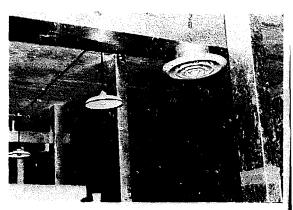
Incoming air diffusers and exhaust stacks passing through the ceiling. Photo courtesy of Canadian Beekeeping.
