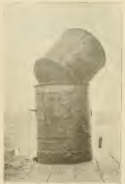
ORIGINAL CAPPING CAN WITH STRAINER REMOVED
