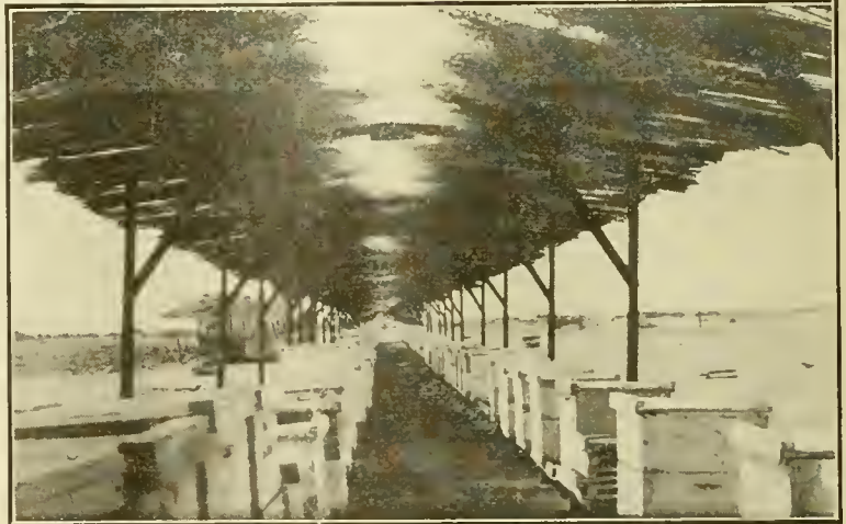
NO. 1.—LOOKING DOWN THROUGH A "RAMADA"
