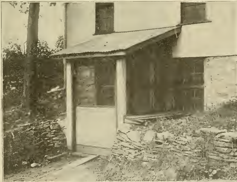
A SCREENED ENTRYWAY PREVENTS THE BEES FROM GETTING INTO THE EXTRACTING HOUSE
