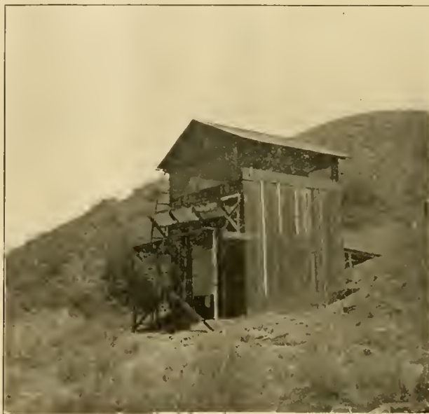
MR. PLEASANTS' TWO-STORY EXTRACTING HOUSE
