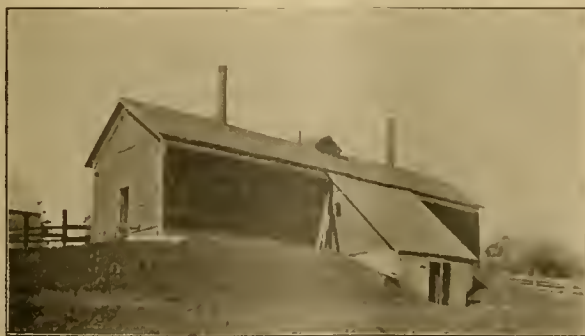
Capt. Hetherington's new Bee-Cellar. Ventilators are large and open all the time. Also openings in the floors over the bees which are open except in the coldest weather. He believed in abundant ventilation for bees.
