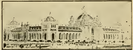
MANUFACTURES AND LIBERAL ARTS BUILDING—PAN-AMERICAN.
