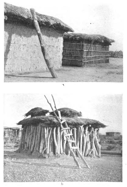
Fig. 29. a Old-time Ladder for filling Pima Granary on House Top; b, Storage House with Two Granaries and Modern Ladder.
