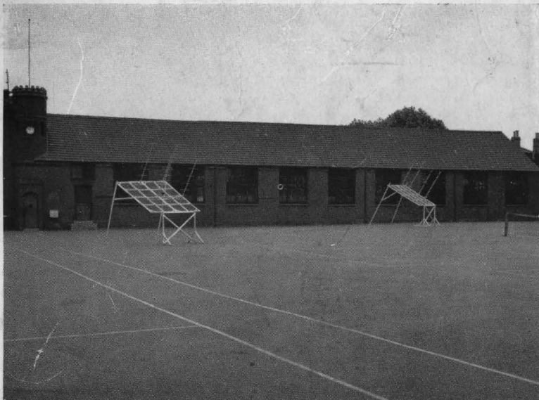
PLATE 4. Arrays of Yagis built by F. W. Hyde in the playground of the Salesian College, Battersea.
