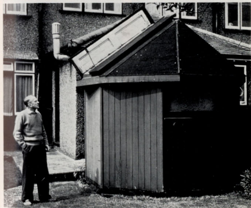
7. Observatories. Above , Patrick Moore's dome, the whole upper section of which revolves. Below , W. M. Baxter's solar observatory with a revolving roof.
