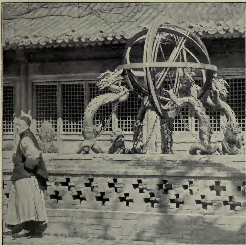
Fig. 95.—Armillary Sphere (an ancient astronomical measuring instrument) at Peking.
