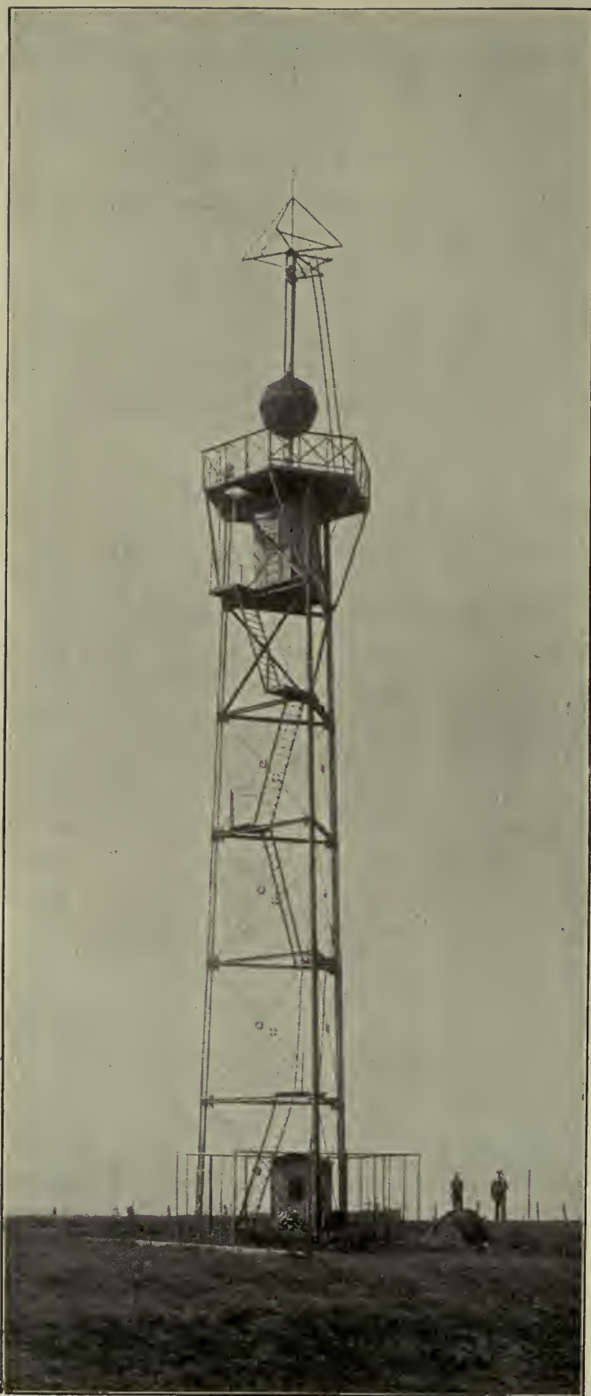
Fig. 90.—Time-ball at Wilhelmshaven.
