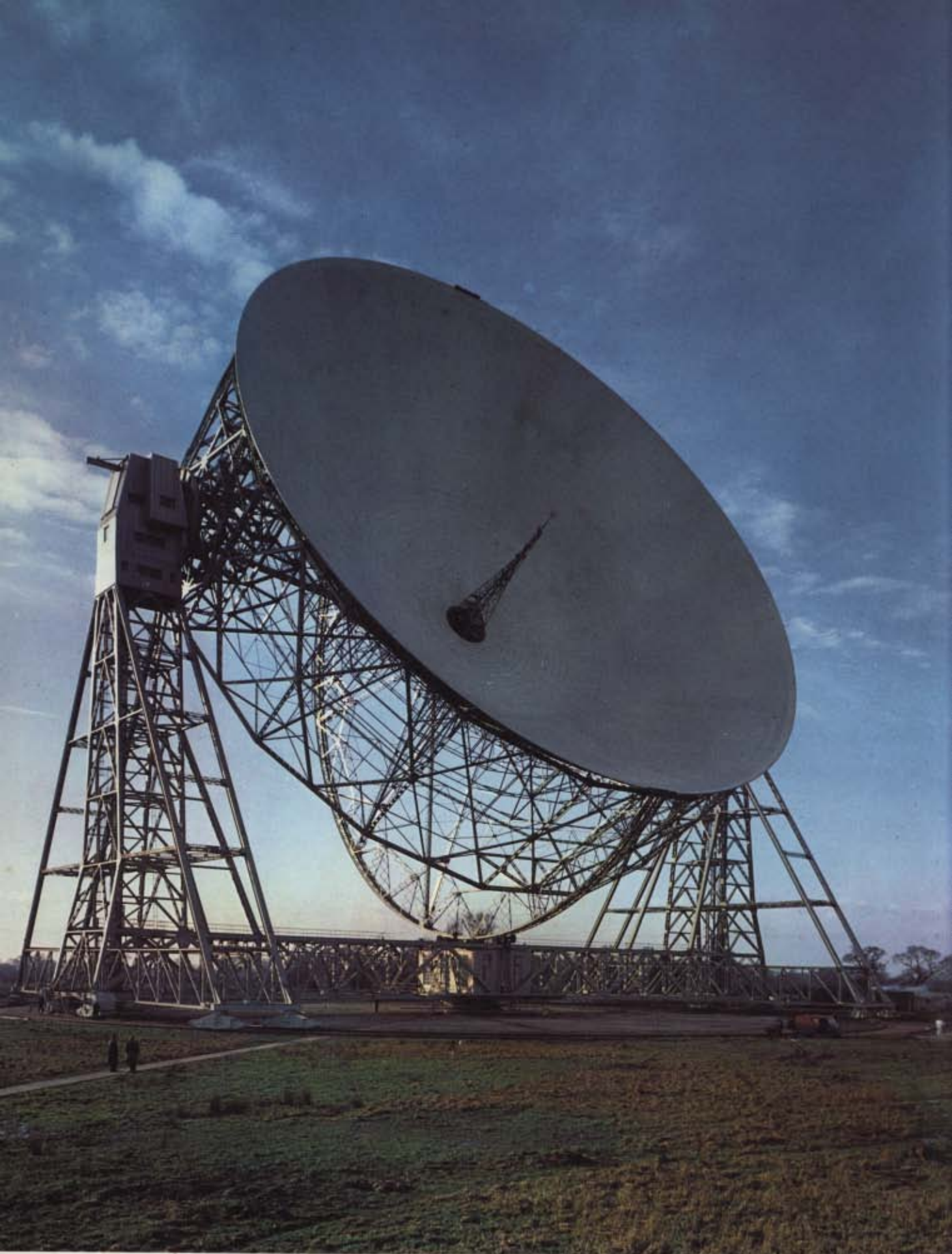
THE 250-FOOT RADIO TELESCOPE OF THE UNIVERSITY OF MANCHESTER, which was opened at Jodrell Bank, in Cheshire, in 1957. It is the largest 'dish'-type radio telescope in the world, and is designed for automatic following of celestial objects across the sky. It is made of steel, and weighs 2,000 tons
