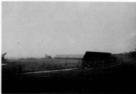
PULKOVO RADIO TELESCOPE. One of the Russian radio telescopes at Pulkovo Observatory, Leningrad. Its main feature is a 'rail' aerial of 90 separate sheets; it has high resolution, and works at a wavelength of 2 to 5 c.m. Photograph by Patrick Moore, 1960
