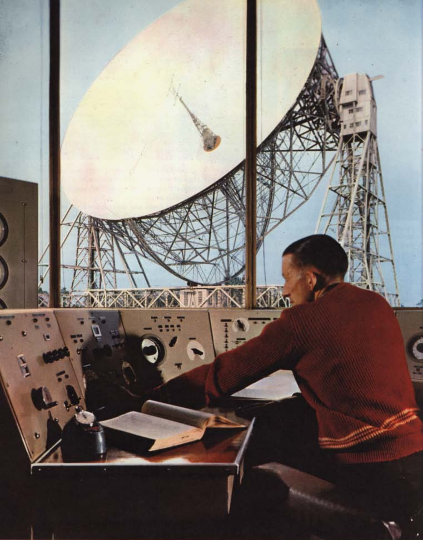
THE JODRELL BANK RADIO TELESCOPE, viewed from the control desk. As well as recording radio waves from space, the telescope has been used to track the various artificial satellites and space-probes launched since 1957
