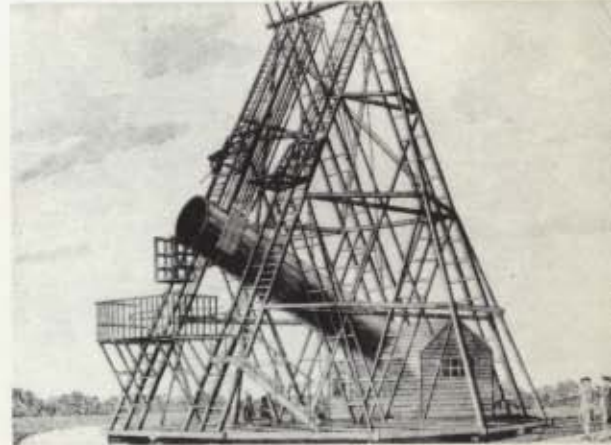
HERSCHEL'S 40-FOOT REFLECTOR, with its scaffolding
