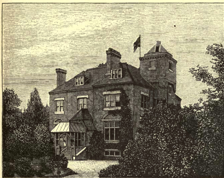
NORTHFIELD GRANGE, EAST-BOURNE : EXAMPLE OF AN OBSERVATORY BUILT AS PART OF A DWELLING-HOUSE.
